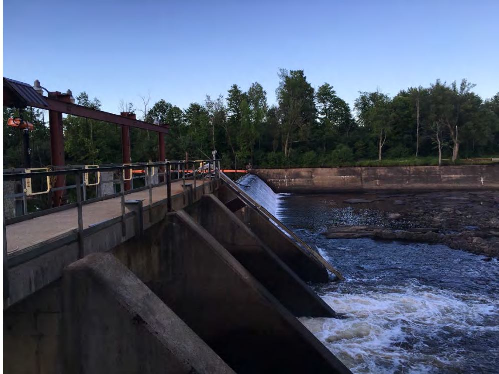
Spillway, Stoplog Structure and Upstream Eel Passage Structure
