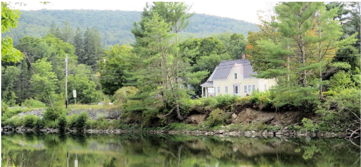
Photo 3-8 Slumping Soils Immediately Upstream of Stone Rip-rap Installations on U.S. Route 4 in August 2024 (GMP 2024)
