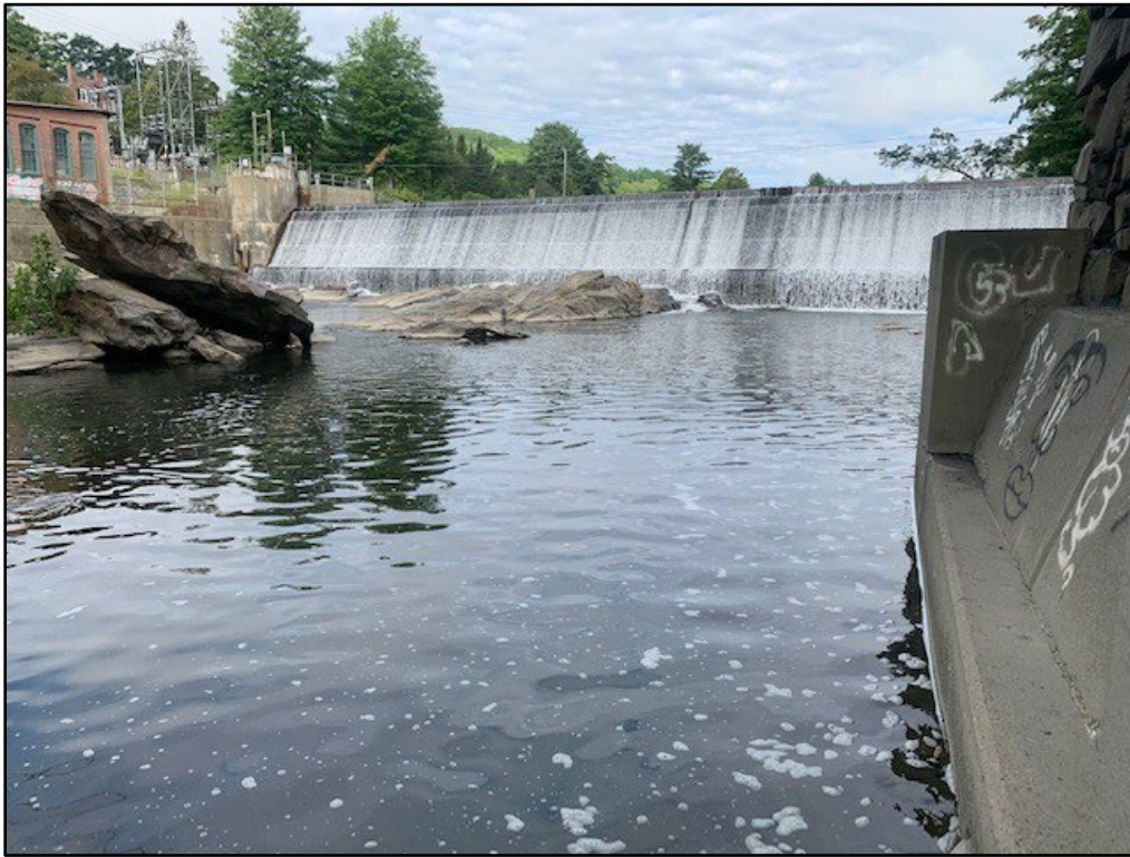
Photo 3-1 Pool Habitat within the Bypassed Reach Directly below the Dam
