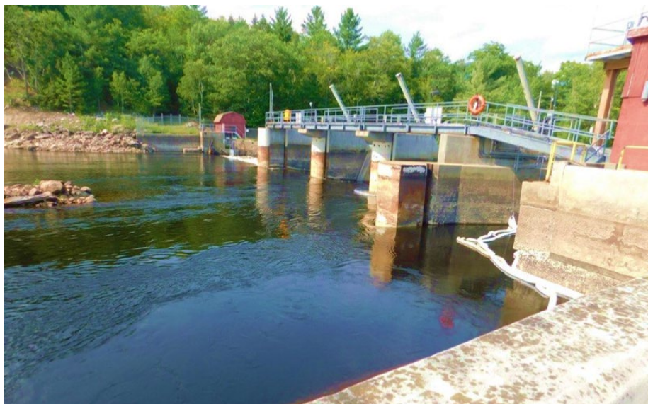
Figure 2 – Shelburne Project on the Androscoggin River in Shelburne, Coos County, NH.
