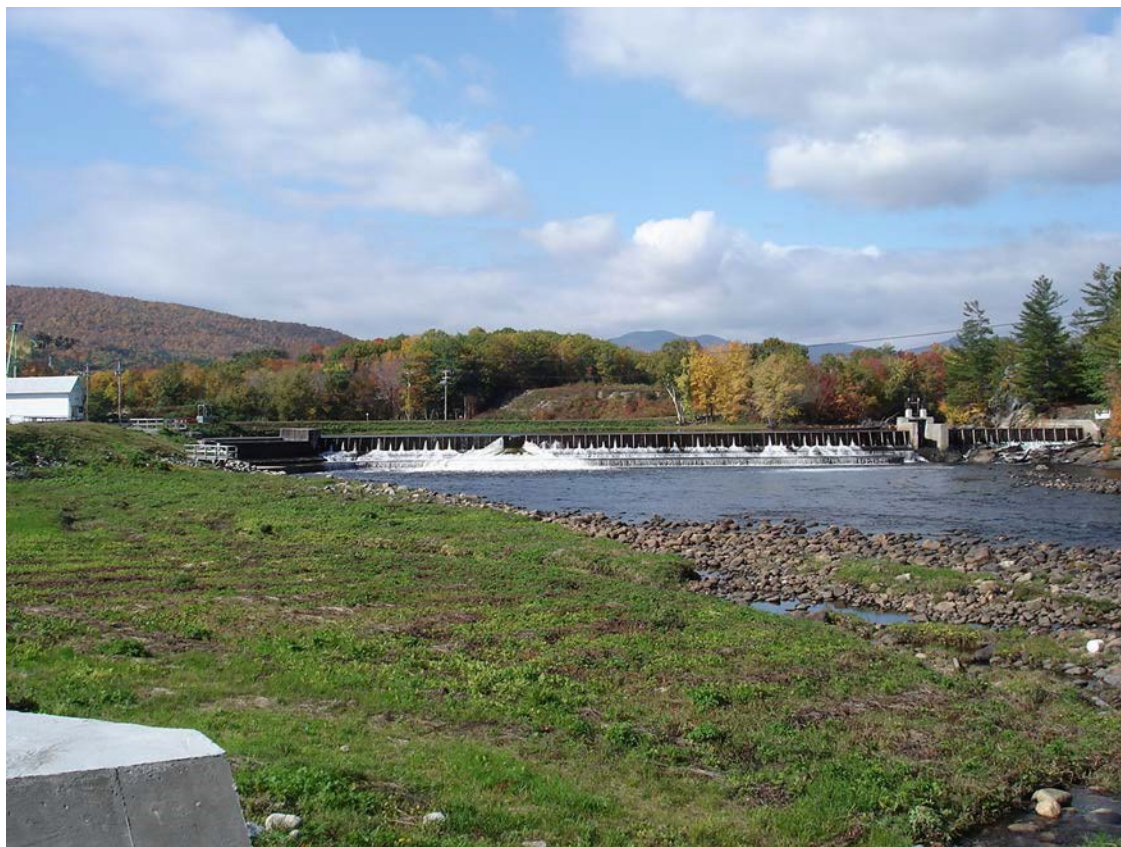
Figure 2 – Gorham Project on the Androscoggin River in Gorham, Coos County, NH.
