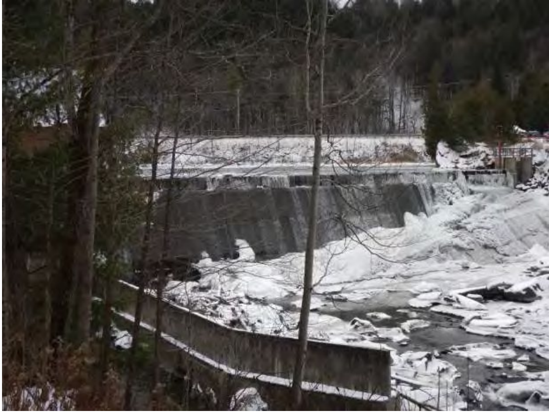
Photo G-3. View of the Winooski 8 Dam with a 1-inch spill flow over the dam, minimum flow unit off (11/18/2019). Source: license application.
