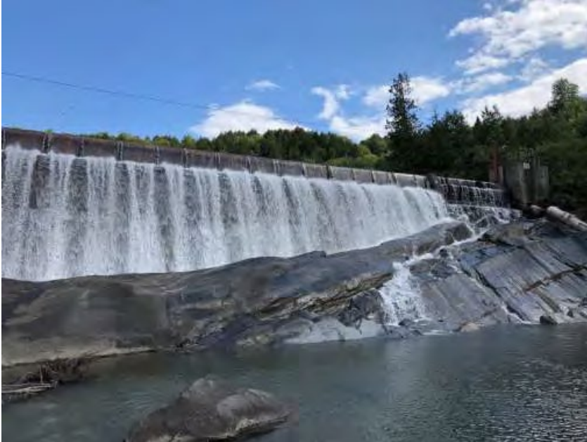
Photos G-7 and G-8. View of the Winooski 8 Dam with a 2.1-inch spill flow over the dam, minimum flow unit on (8/30/2019). Source: license application.
