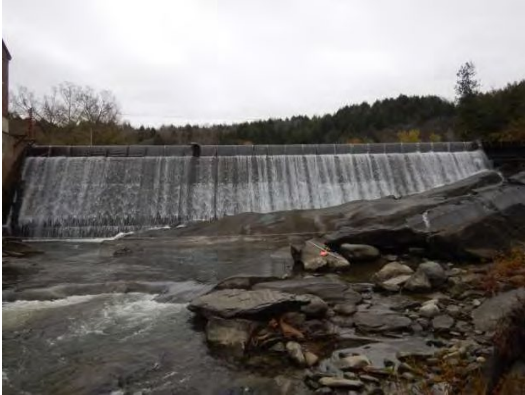
Photo G-5. View of the Winooski 8 Dam with a 0.5-inch spill flow over the dam, minimum flow unit on (10/22/2019). NOTE: Flows could not be maintained stable during this flow measurement, but the picture has been included and compares reasonably well with the 1.2-inch spill photograph. Source: license application.
