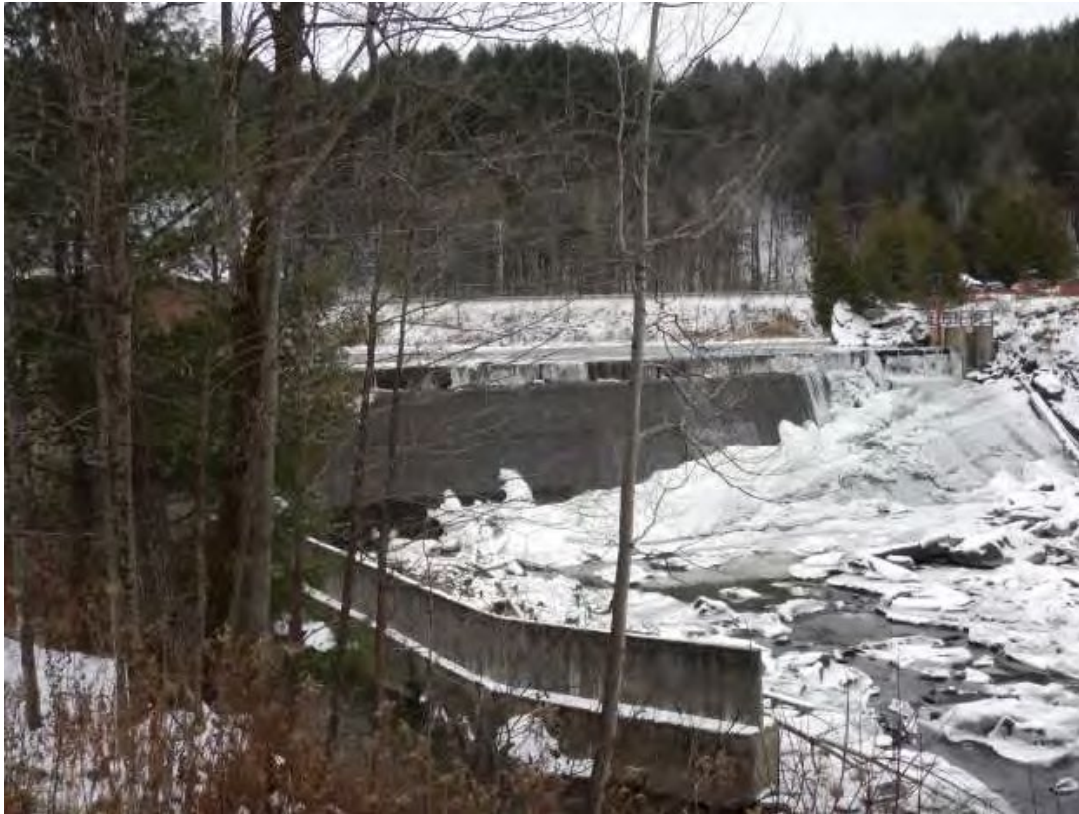
Photo G-1. View of the Winooski 8 Dam with a 0.5-inch spill flow over the dam, minimum flow unit off (11/18/2019). Source: license application.
