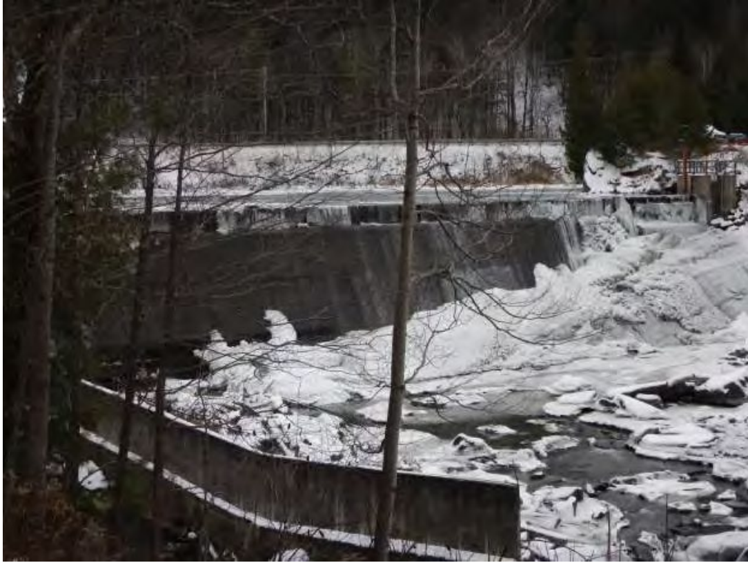
Photo G-2. View of the Winooski 8 Dam with a 0.75-inch spill flow over the dam, minimum flow unit off (11/18/2019). Source: license application.
