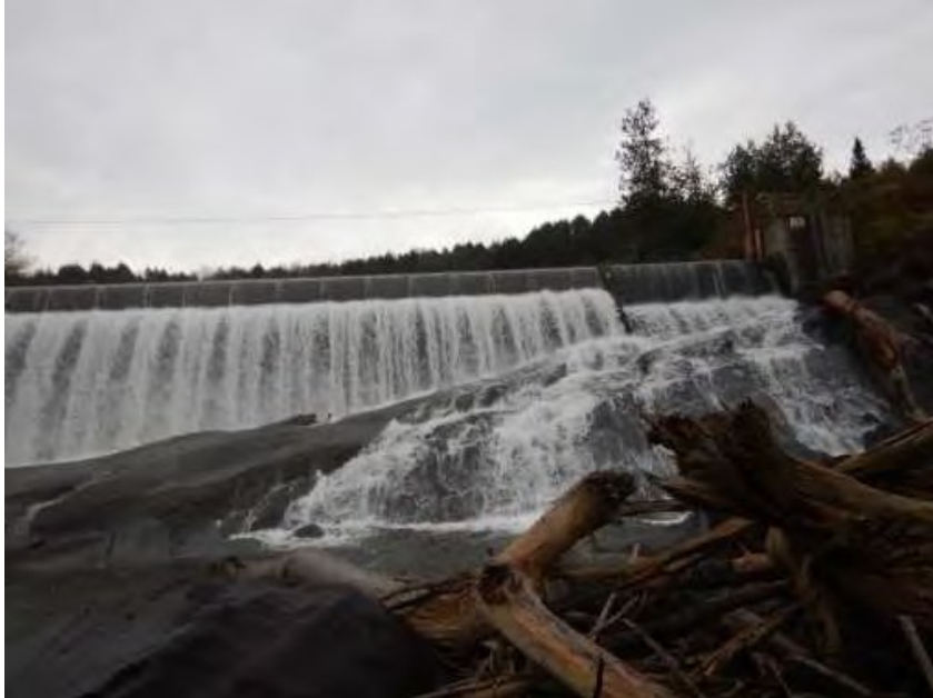
Photos G-9 and G-10. View of the Winooski 8 Dam with a 3.7-inch spill flow over the dam, minimum flow unit off (10/22/2019). Source: license application.
