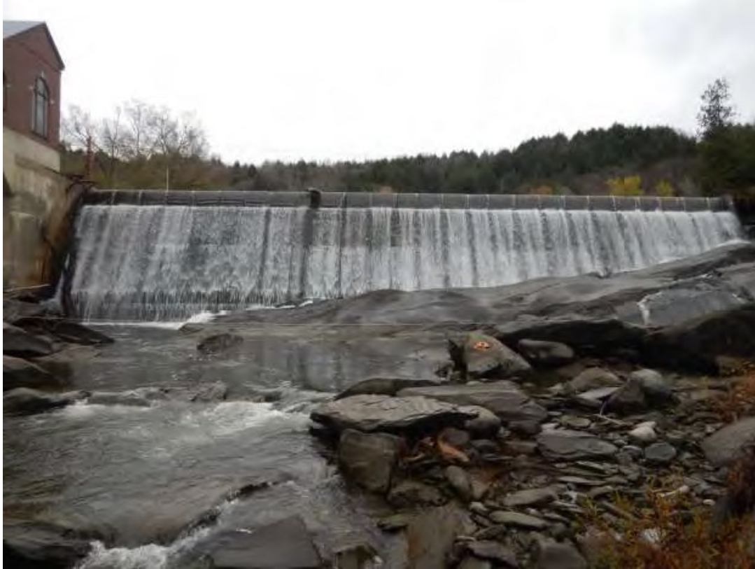
Photo G-6. View of the Winooski 8 Dam with a 1.2-inch spill flow over the dam, minimum flow unit off (10/22/2019). Source: license application.
