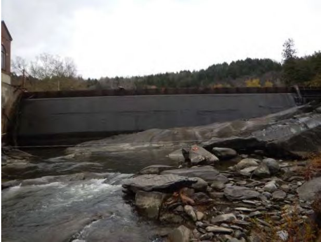
Photo G-4. View of the Winooski 8 Dam with a 0-inch spill flow over the dam, minimum flow unit on (10/22/2019). Source: license application.
