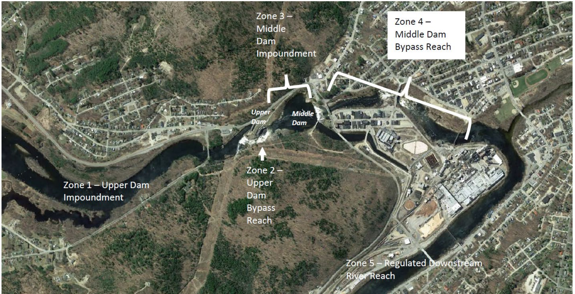
Figure 1-1 Zones of Effect for the Rumford Falls Hydroelectric Project Based on the 2019 LIHI Application
