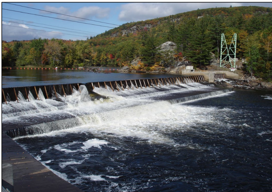
Photo 3.2 Gorham Dam and Minimum Flow Release into Upper Section of Bypass Reach
