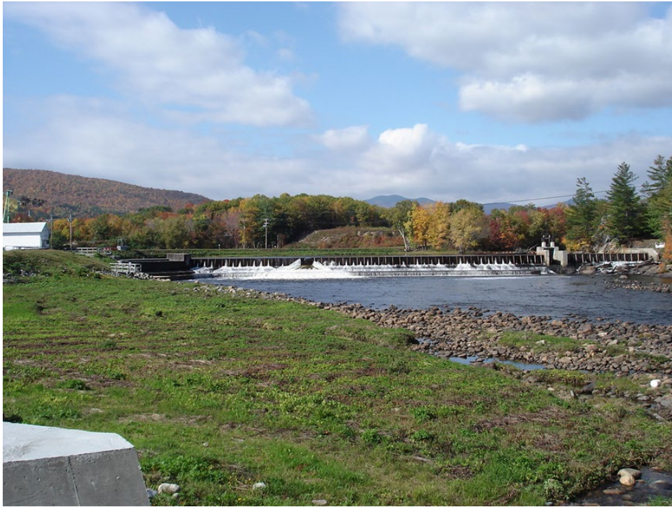
Photo 2.1 Gorham Project Dam
