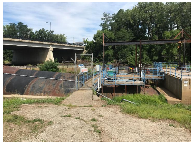
Figure 4. Powerhouse and Penstocks
