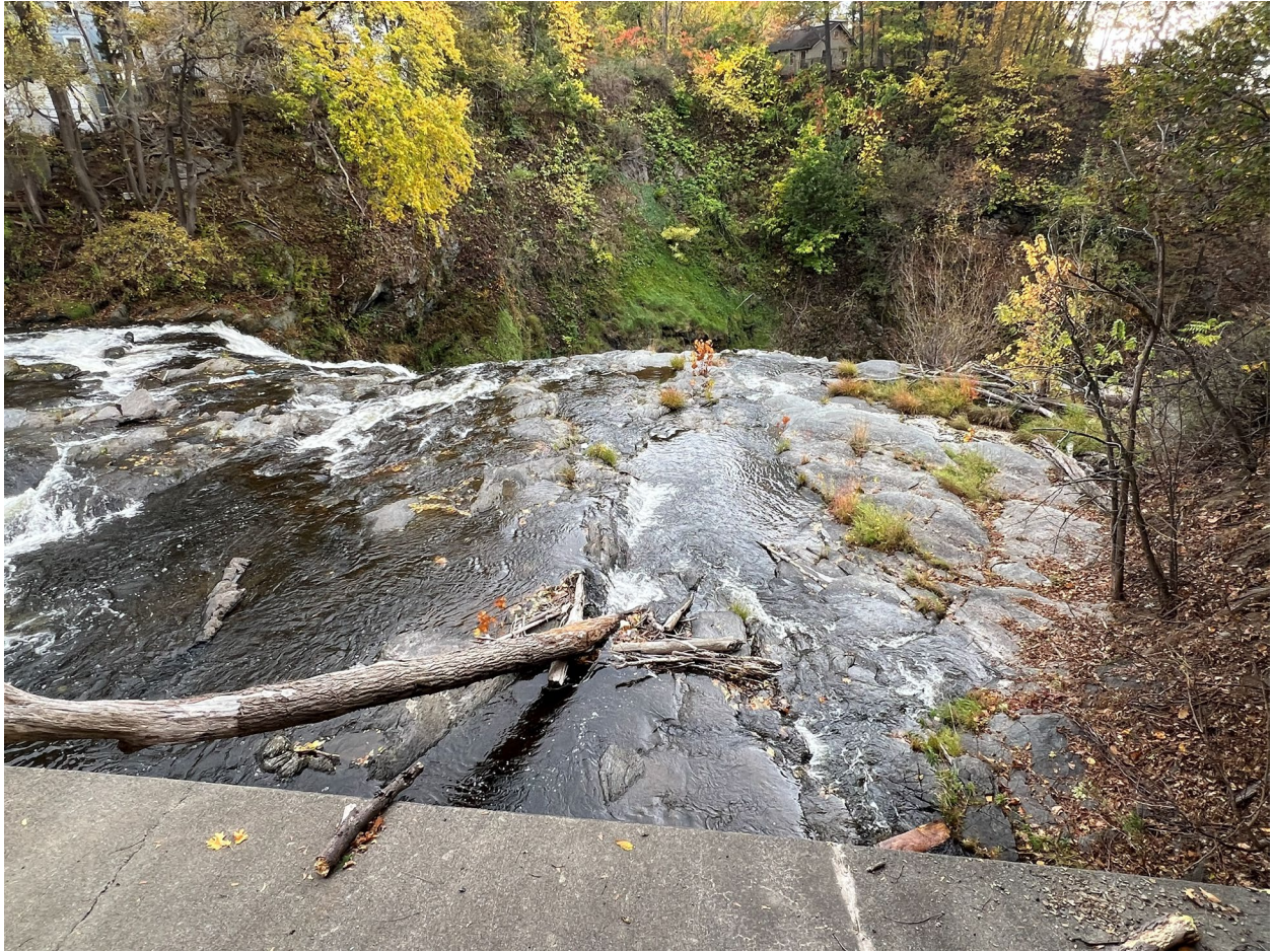
Figure 8. Mt Ida Dam Tailrace
