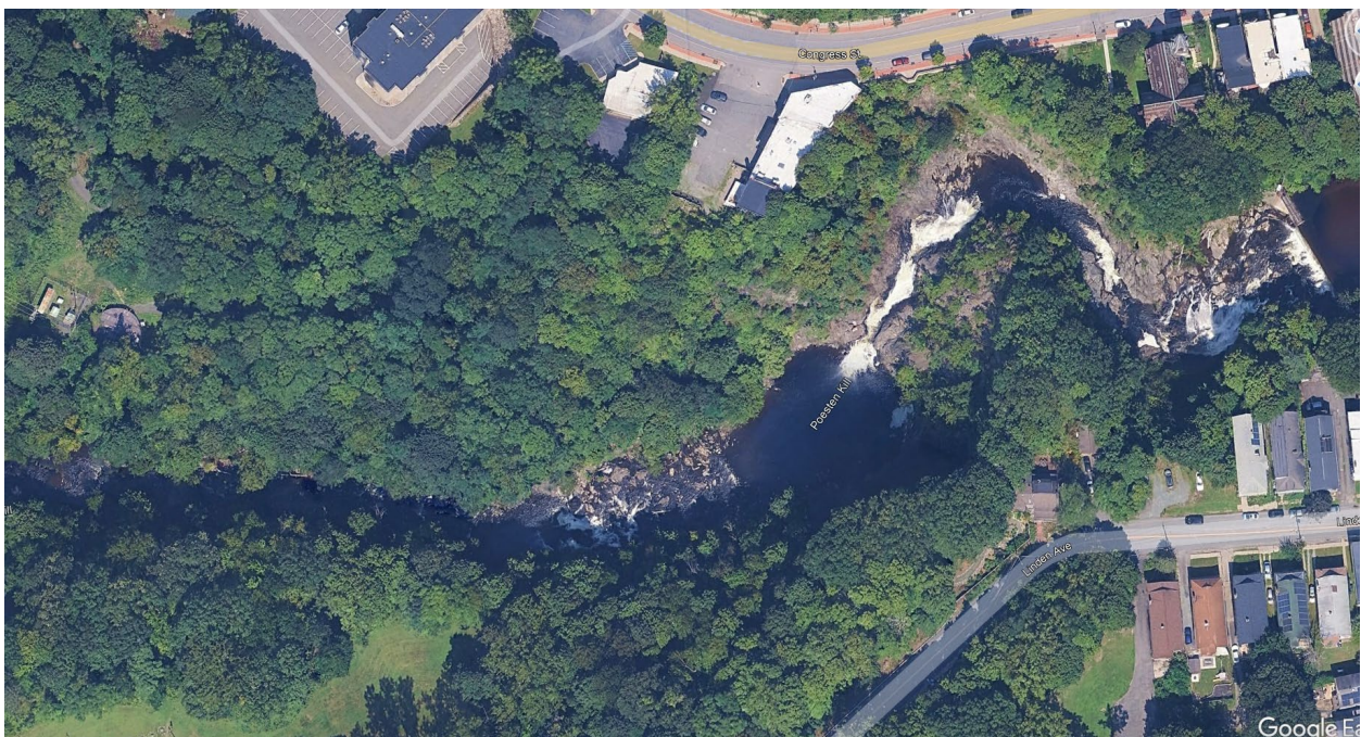
Figure 3. Mt Ida Project Facilities (Bypass Reach)
