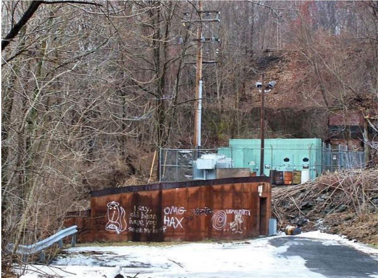
Figure 5. Mt Ida Powerhouse (Exterior)
