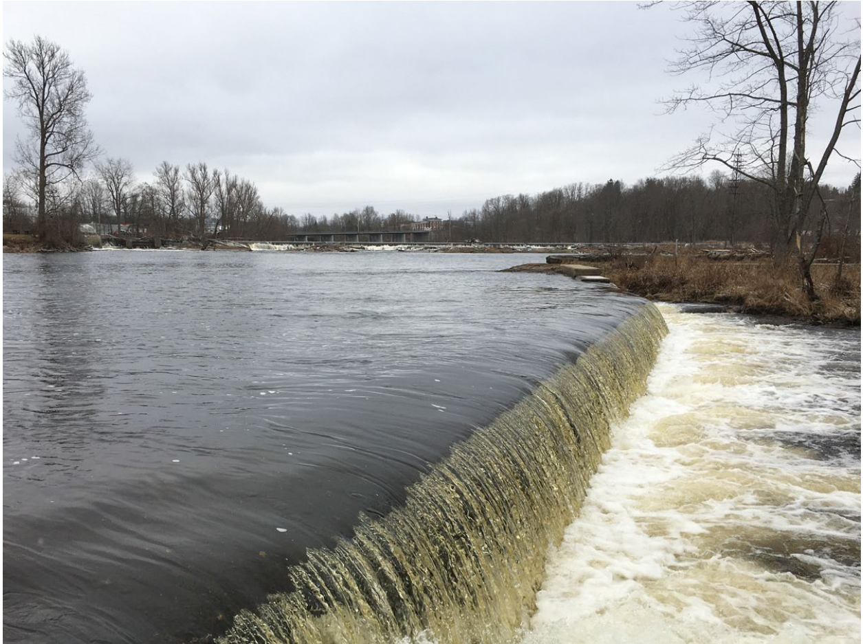
Figure 2. Tannery Island Project Facilities (Impoundment, Tannery Island Dam “B” Spillway and Bypass Reach)
