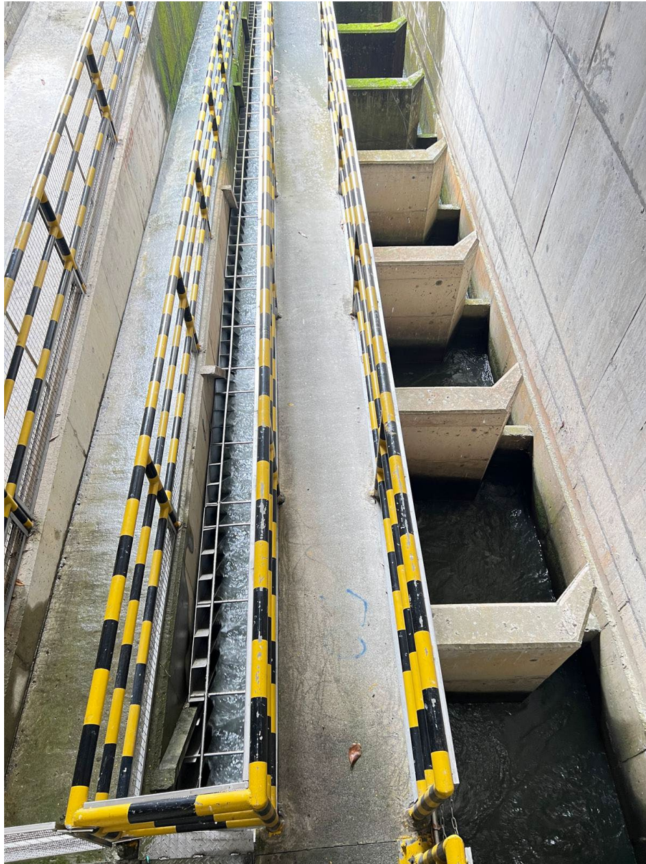
Figure 4. Ma'an Dam Fishways – Denil (at left) and Pool/Weir (at right)
