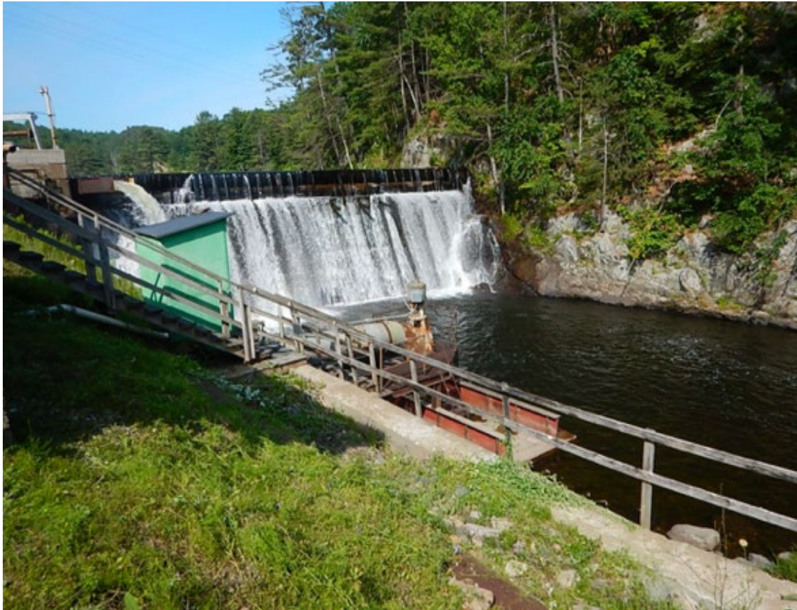
Figure 3. Newbury Project dam, spillway, and other features.
