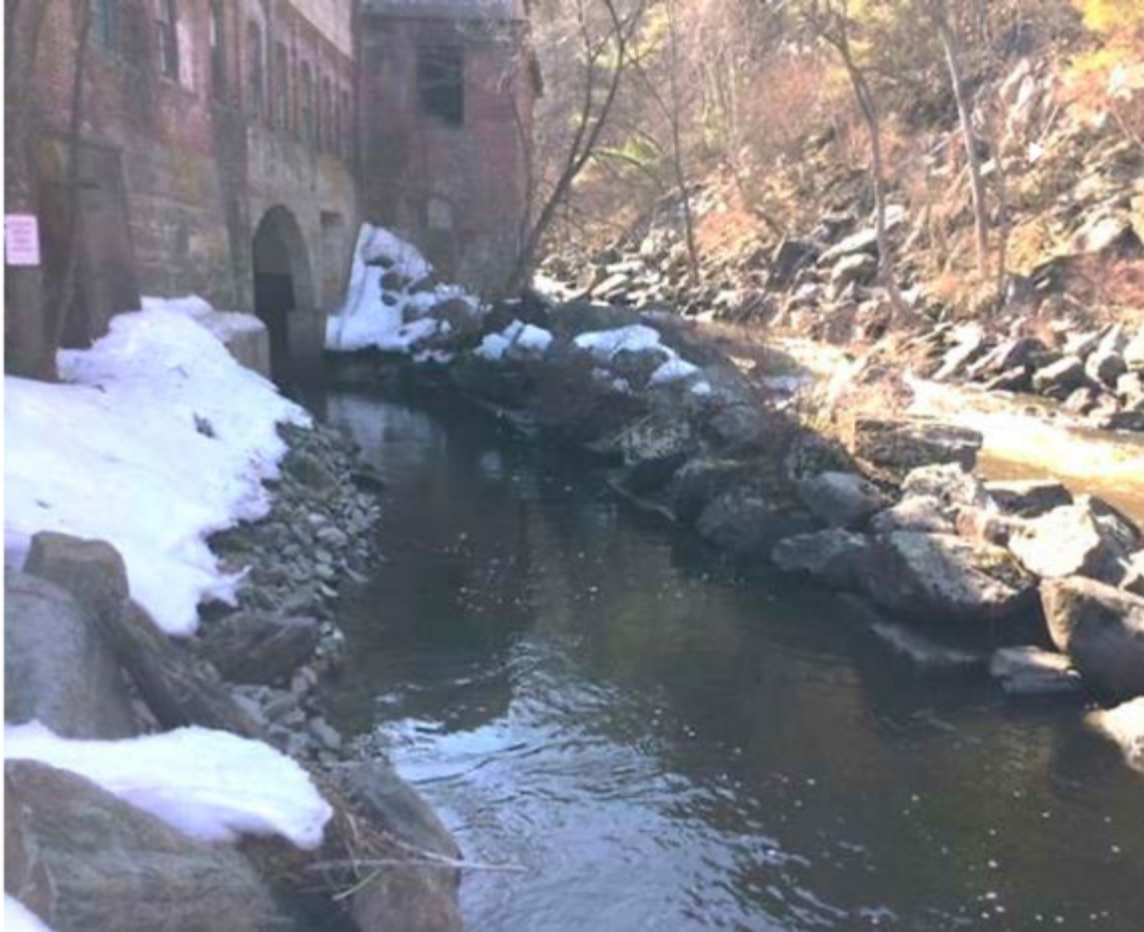
Figure 5. Newbury Project Tailrace.
