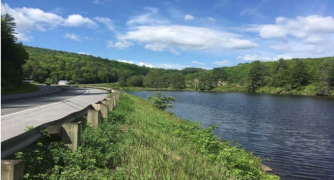
Figure 13. Project Reservoir bordered by U.S. Route 302 to the south.
