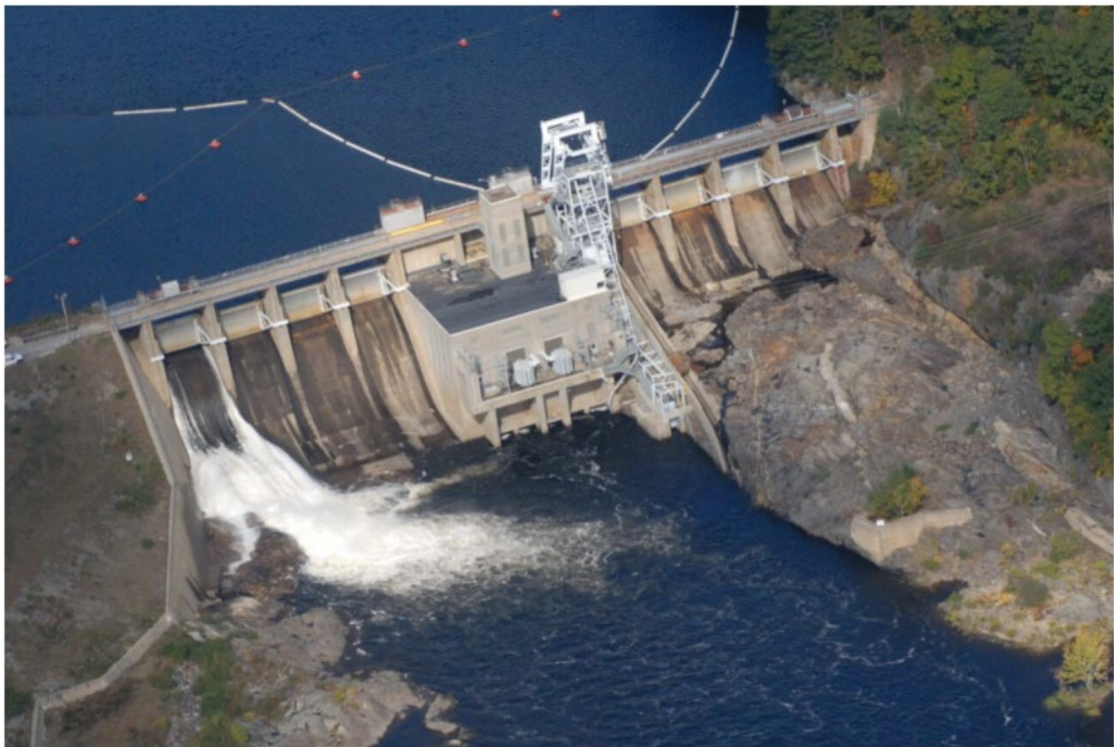
Figure 2. – Photograph of Skelton Project (aerial) showing the Impoundment, Dam, Powerhouse, and Tailrace.
