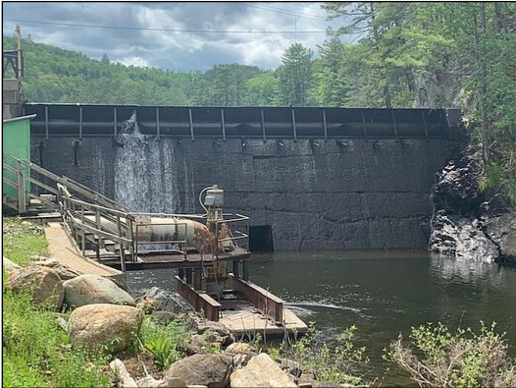
Photo 10 Flow Release 1 (Leakage)
