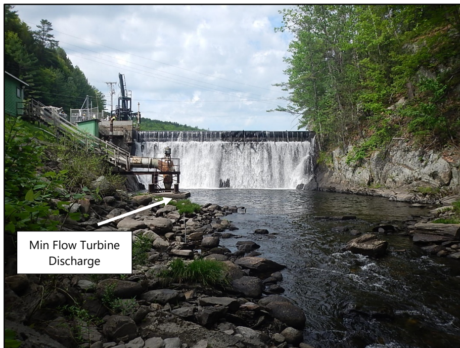
Photo 1 Newbury Dam, Minimum Flow Turbine, Plunge Pool, and Upper Section of the Bypassed Reach
