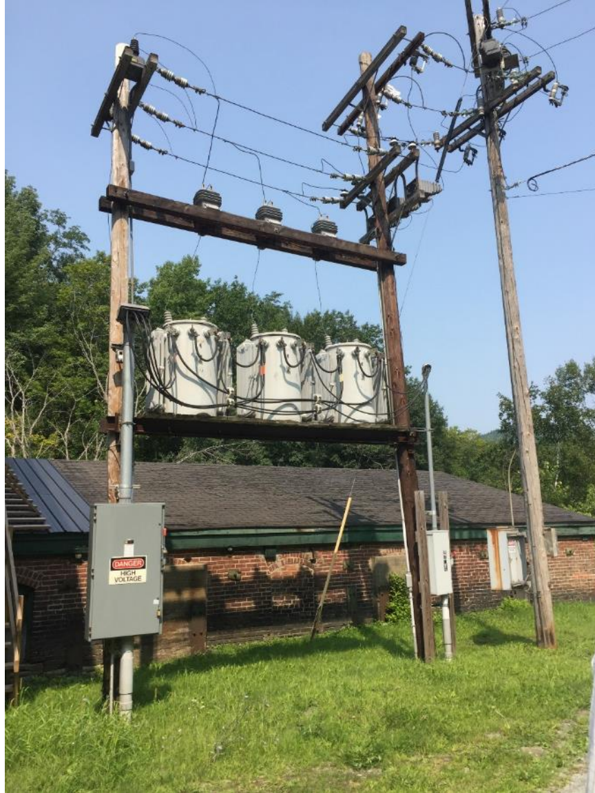
Photo 2.10 Three Step-Up Transformers
