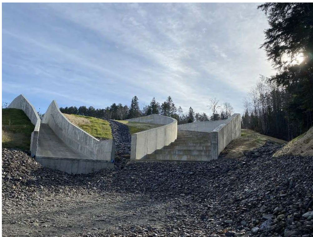
Figure 4. Marshfield Dam Service Spillway (left) and Emergency Spillway (right)
