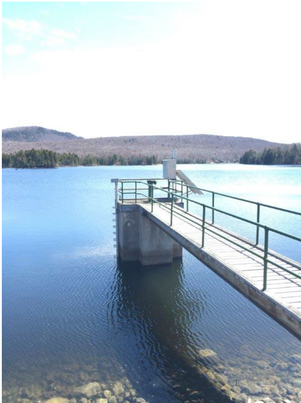
Figure 5 Peacham Pond Outlet Works and Access Bridge
