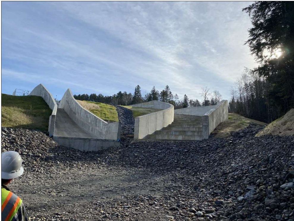
Figure 10 Marshfield Emergency Spillway (right), and Service Spillway (left), and Plunge pool (foreground)
