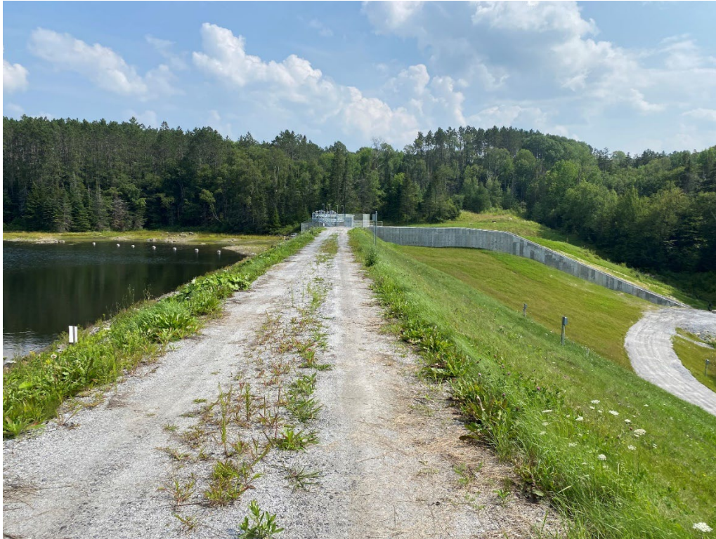
Figure 8 Marshfield Earthfill Rolled Dam
