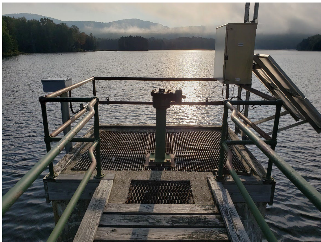
Figure 6 Peacham Pond Outlet Works, viewed from the Access Bridge
