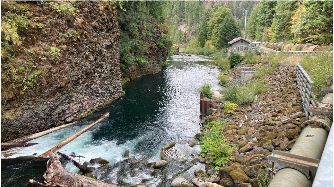
Photo 34. Looking downstream (northwest) at the Soda Springs bypassed reach (ZOE 11). Fish screened from diversion are returned to the river via the pipe at the bottom right of frame. The Fish Evaluation Building is seen on river-right in the middle distance.
