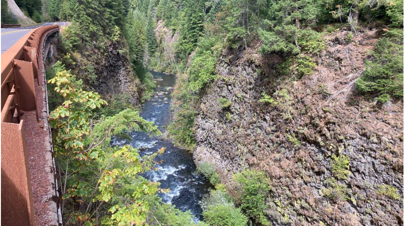
Photo 45. Looking downstream (north) from the Highway 138 bridge over the lower Fish Creek bypassed reach (ZOE 18; left of frame) confluence with the Slide Creek bypassed reach of the North Umpqua River (ZOE 8).
