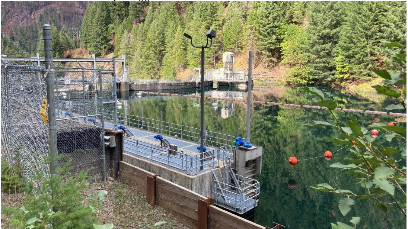
Photo 32. Looking northeast at Soda Springs Reservoir (ZOE 10). Fish ladder exit gates are seen in the lower middle of frame. Soda Springs dam crest and the north intake tower are seen in the middle distance.
