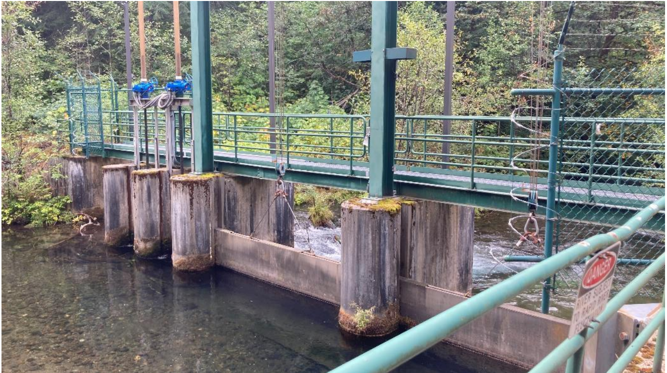
Photo 41. Looking downstream (southwest) at the Clearwater Reconnect facility and the Clearwater No. 2 bypassed reach (ZOE 16).
