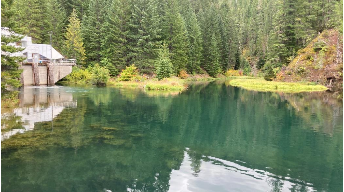
Photo 11. Looking upstream at the lower Lemolo No. 1 bypassed reach (ZOE 2) where it enters the Lemolo No. 2 impoundment (ZOE 3). The Lemolo No. 1 powerplant and tailrace are seen on the left of frame.
