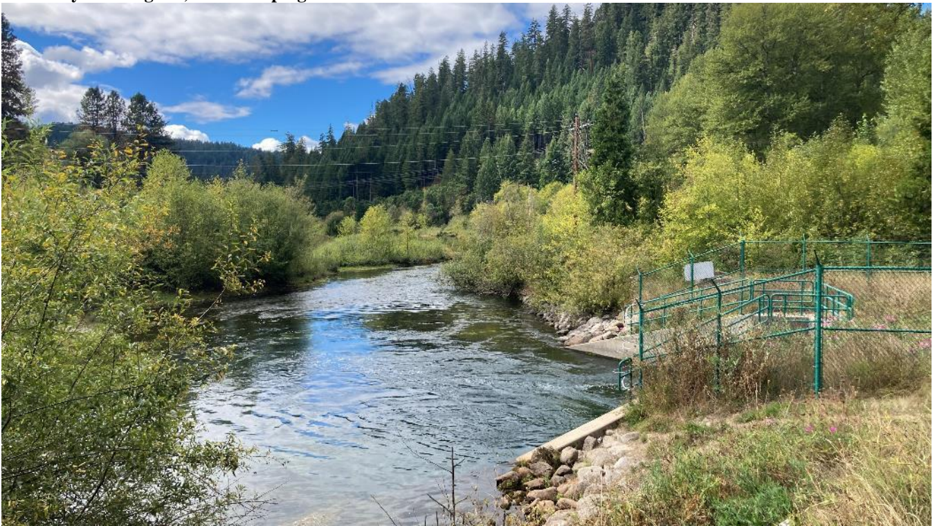
Photo 16. Looking downstream (west) at the discharge of the Lemolo No. 2 bypassed reach (ZOE 4) into upper Toketee Reservoir (ZOE 5). The Lemolo No. 2 reroute pipeline discharge is seen at the right of frame.
