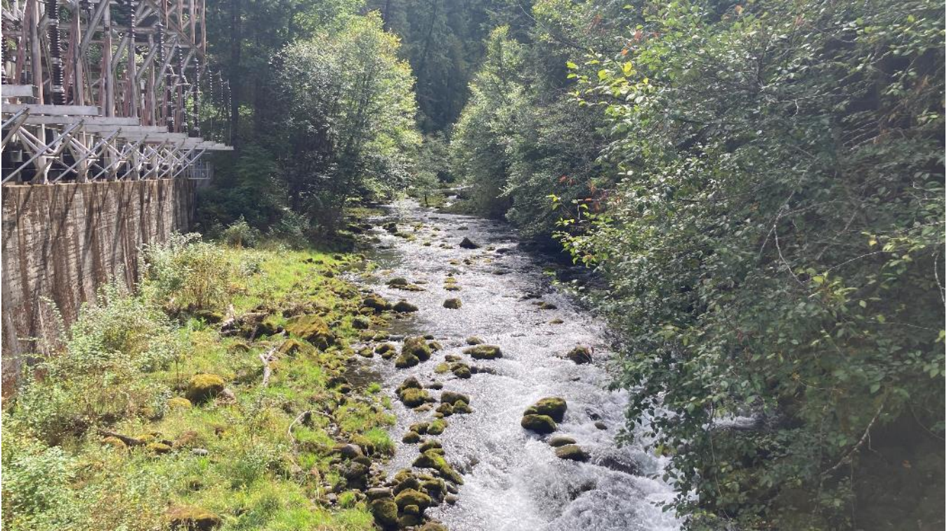
Photo 25. Looking upstream (south) at the lower Toketee bypassed reach of the North Umpqua River (ZOE 6). The Toketee powerhouse substation is seen at left of frame.
