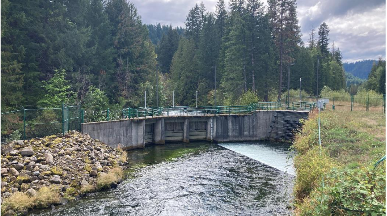
Photo 15. Looking south at the Lemolo No. 2 reroute structure. Lemolo No. 2 powerplant tailrace flows enter the pipeline at the right of frame, thereby protecting the lower Lemolo No. 2 bypassed reach (ZOE 4; seen at center of frame beyond the gates) from ramping.
