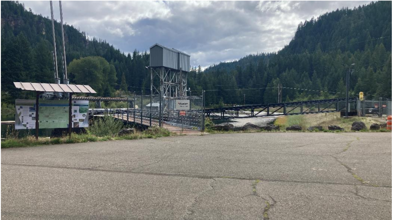
Photo 23. Looking southeast from the right abutment of Toketee Dam at Toketee Reservoir (ZOE 5) and the Toketee waterway intake and trash rake. FPA Part 8 recreational signage is see at left of frame.
