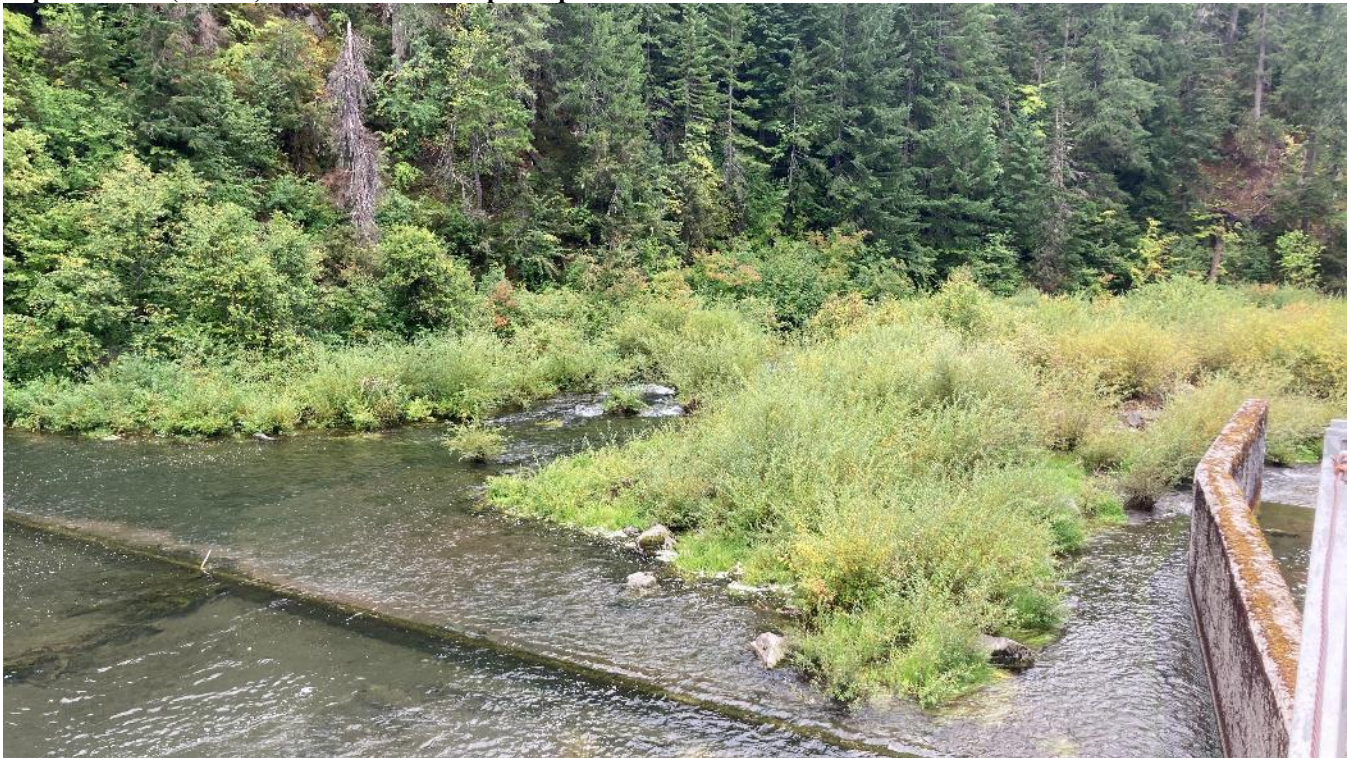
Photo 12. Looking downstream from Lemolo No. 2 dam at the upper Lemolo No. 2 bypassed reach of the North Umpqua River (ZOE 4).
