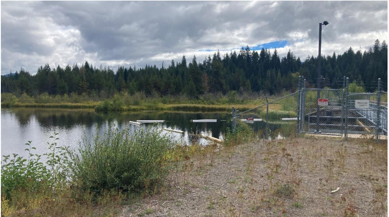
Photo 37. Looking east from the right embankment of Clearwater No. 1 dam at Clearwater No. 1 impoundment (Stump Lake; ZOE 13).
