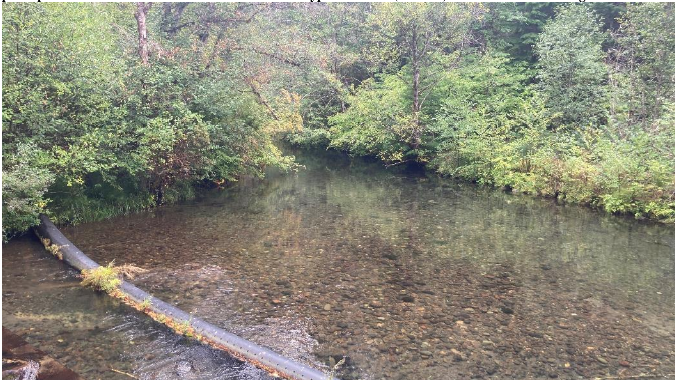
Photo 40. Looking upstream (east) from the right abutment of the Clearwater Reconnect facility at the Clearwater No. 2 bypassed reach (ZOE 16). Flows at left of the boom continue to Toketee Reservoir. Flows to the right of the boom continue downstream of the Clearwater Reconnect facility to the lower Clearwater No. 2 bypassed reach.
