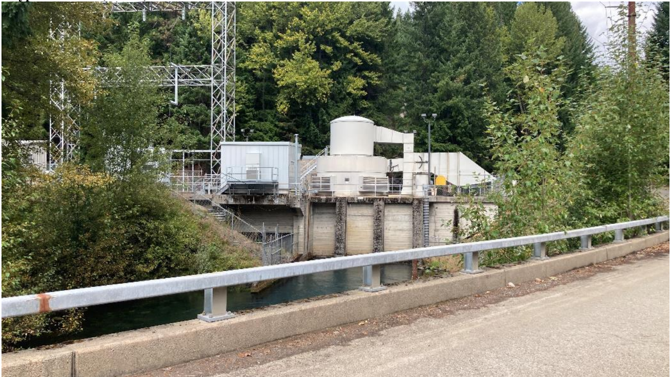
Photo 14. Looking northwest from Forest Service Road 34 at Lemolo No. 2 powerplant.
