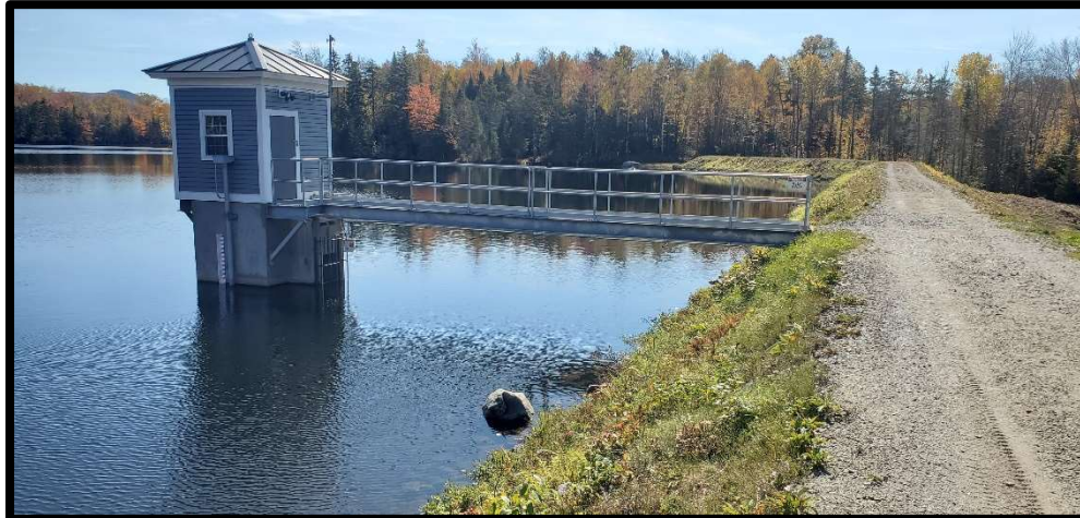
Figure 4: Peacham Pond Outlet Works, viewed from the north
