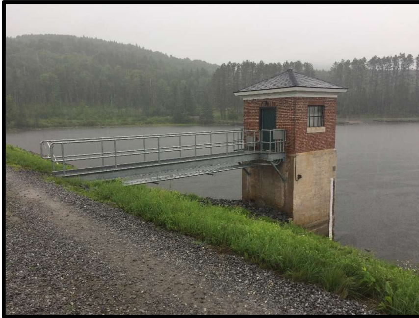
Figure 6: Molly's Falls Reservoir Gatehouse, viewed from the south
