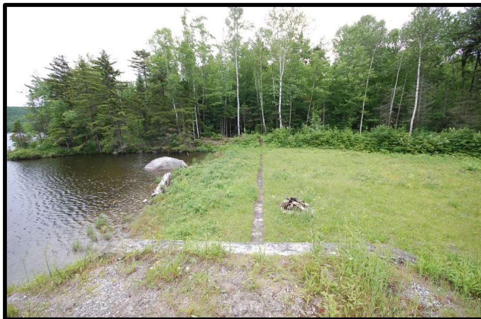
Figure 5: Peacham Pond Spillway, viewed from the north
