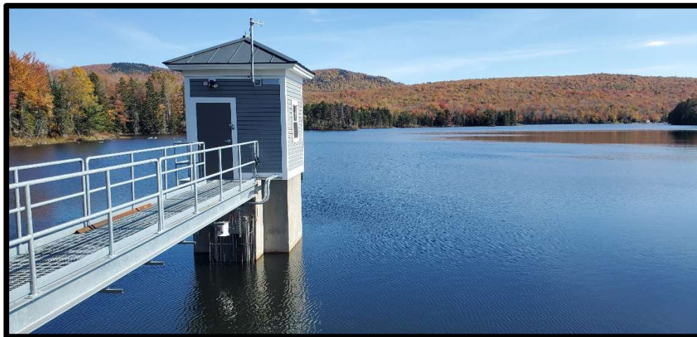
Figure 3: Peacham Pond Outlet Works, viewed from the west Weir visible on face of structure below bridge
