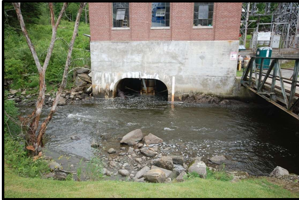
Figure 9: Molly's Falls Powerhouse, viewed from the west
