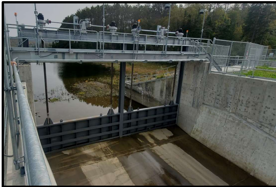
Figure 10: Molly's Falls Reservoir Service Spillway, viewed from the west
