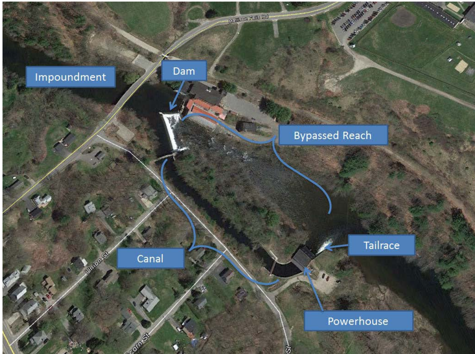
Fig. 2 – Aerial of Project and Key Features
