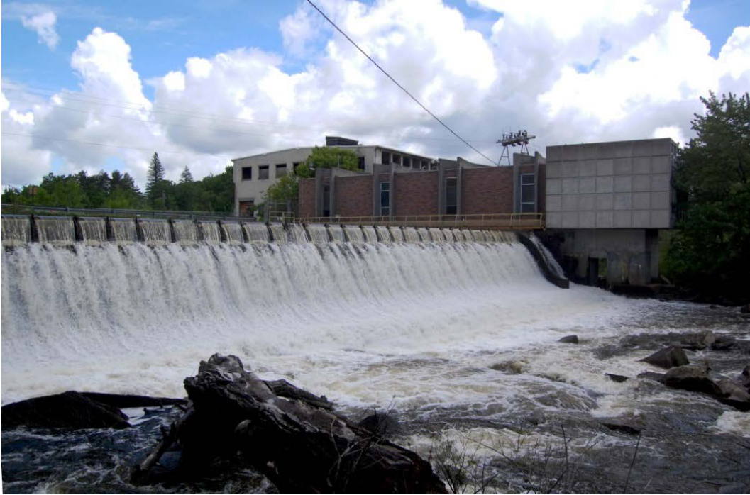
Powerhouse and Spillway
