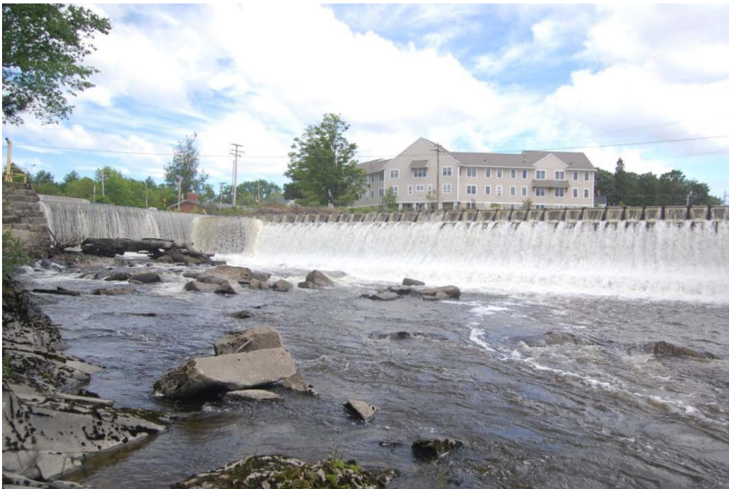
Spillway and Bypass
