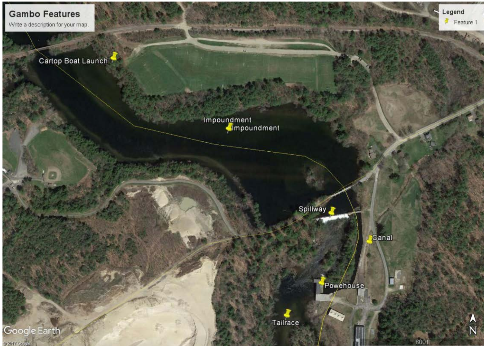
Fig. 2 – Aerial of Project and Key Features
