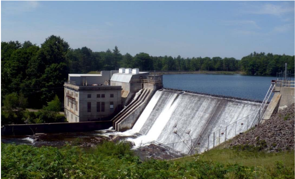
Spillway and Powerhouse
