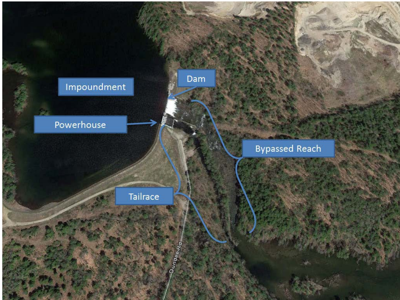
Fig. 2 – Aerial of Project and Key Features
