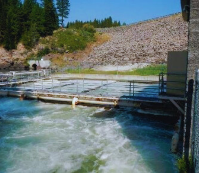
Figure 9. Water discharged from the Island Park project enters this specially designed aeration basin, where it is churned to add oxygen before being released downstream.
