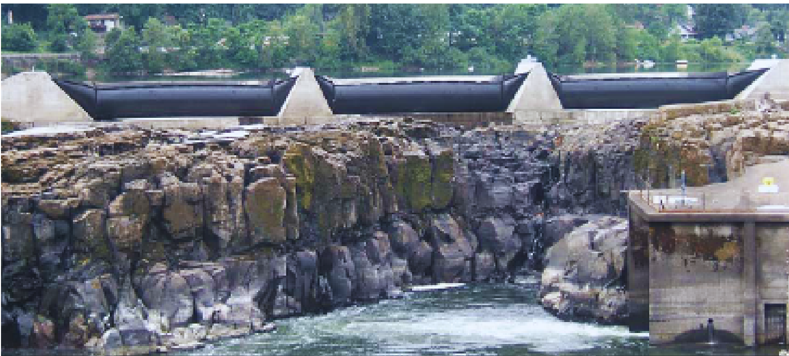
Figure 8. The three inflatable rubber bladders depicted here direct additional water into a deep pool, providing a safe landing for fish that pass downstream over the natural Willamette Falls.
