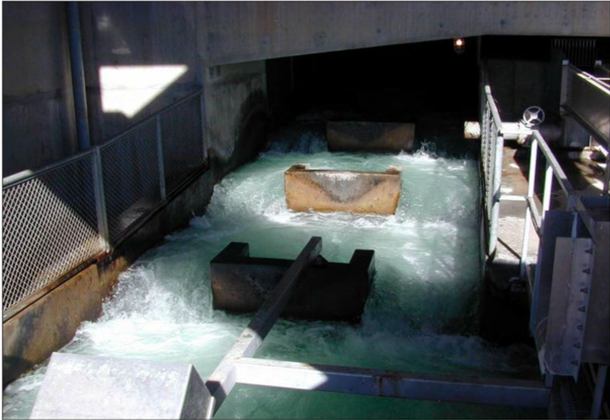
Figure 15. Wells Project adult fish ladder weirs
