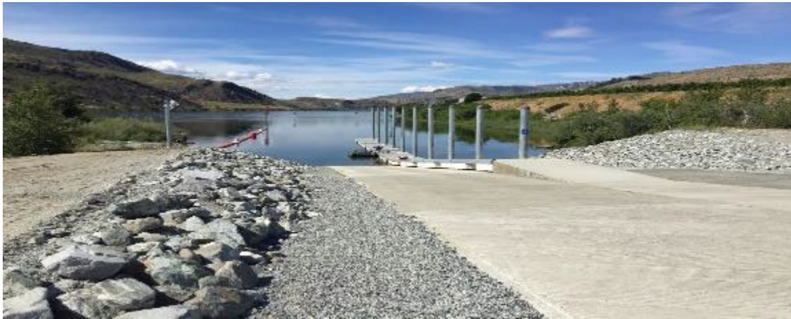
Figure 29. Photo of Carpenter Island Boat Launch one mile downstream of Wells Dam.
