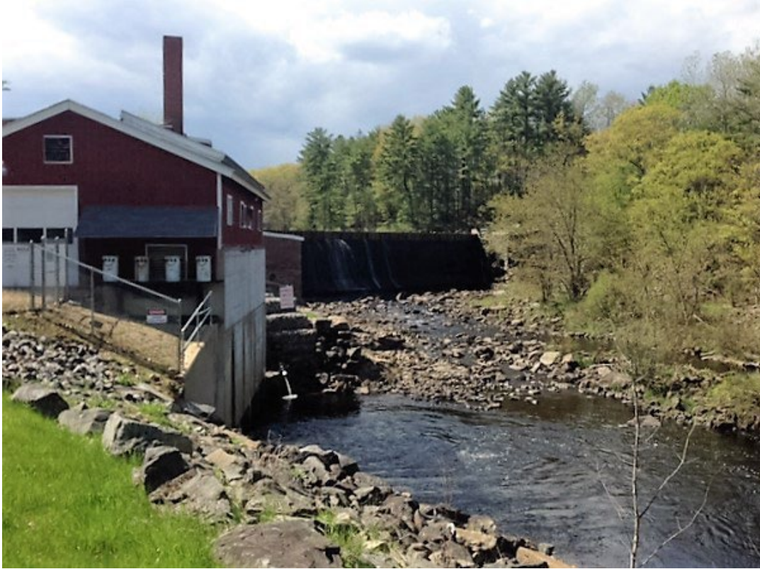
Figure 4 – Powerhouse and Tailrace
