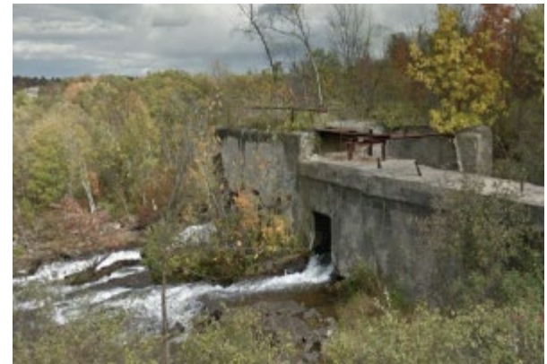
Figure 9-Mill B Dam flow through
