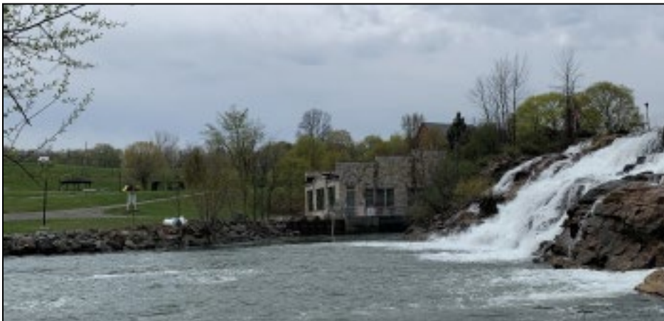
Figure 6-Lower LaChute Powerhouse and Mill F Dam falls
