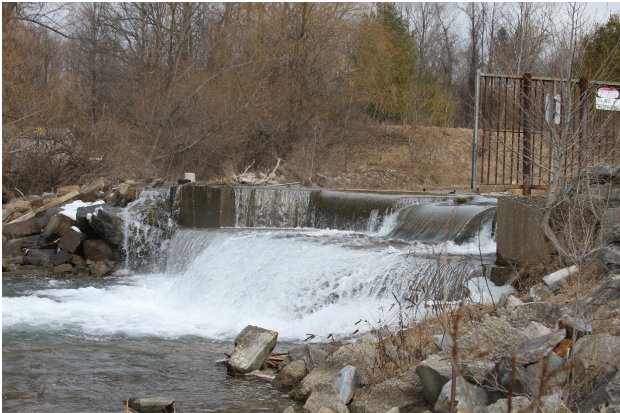
Upper project, C-Mill dam min flow notch from downstream (sized for 30 cfs; any bypass flow over 30 cfs is passed in dam leakage and slight spill)
