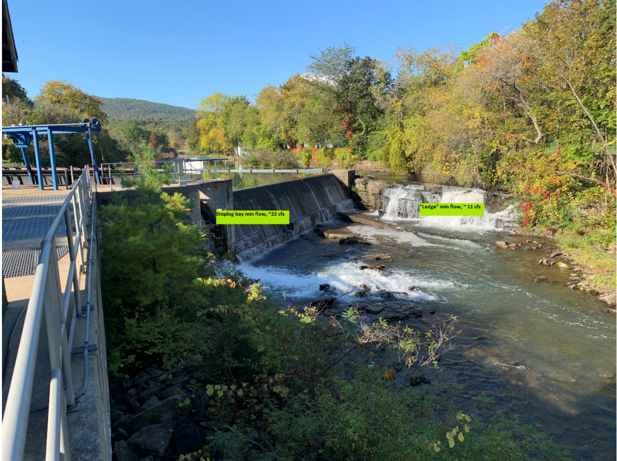
Lower project, ledge and stoplog bay min flow below primary (intake) D-mill dam on left. See also LIHI Stage 1 Application photo 1.6 for view of stoplog bay, from upstream
