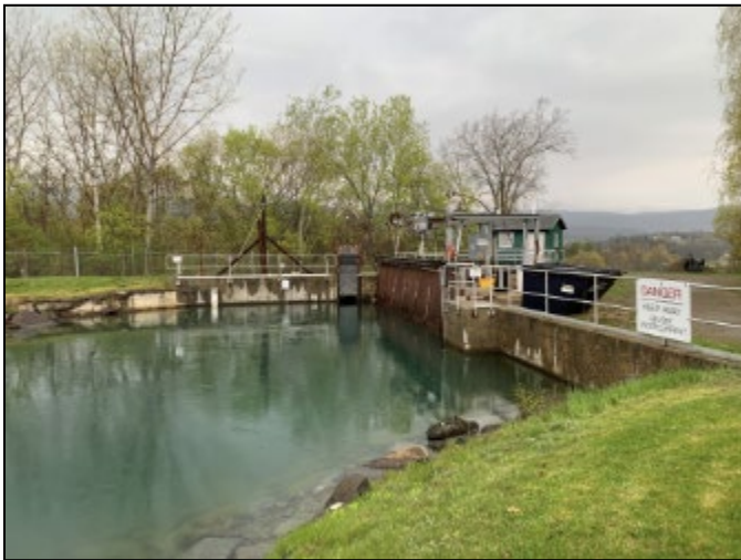
Figure 2-Upper LaChute Intake and Fish Bypass Facility
