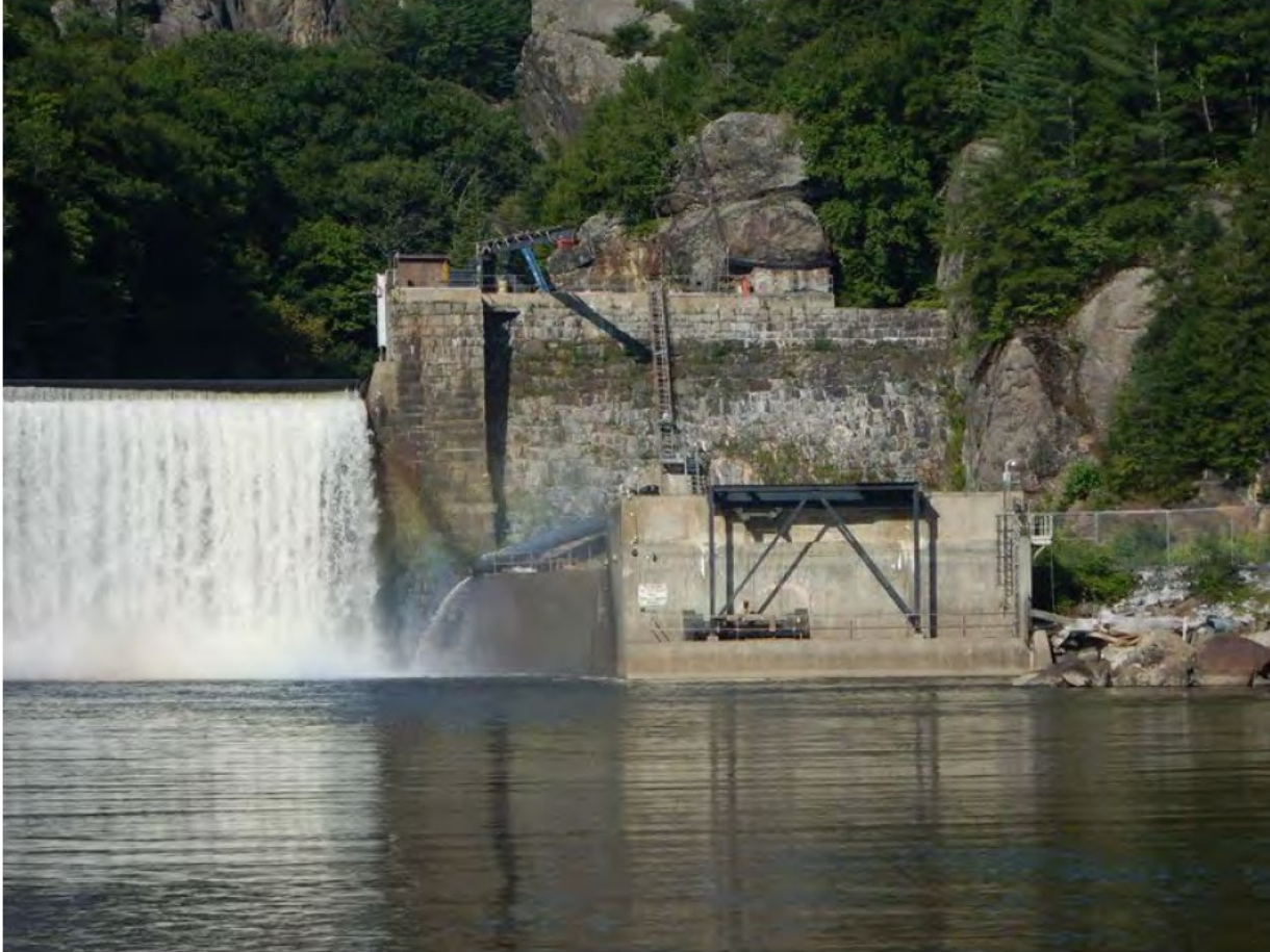
Figure 4. – Photograph of Bolton Falls Project Dam, Bypassed Reach, Powerhouse, Tailrace and Minimum Flow Pipes.
