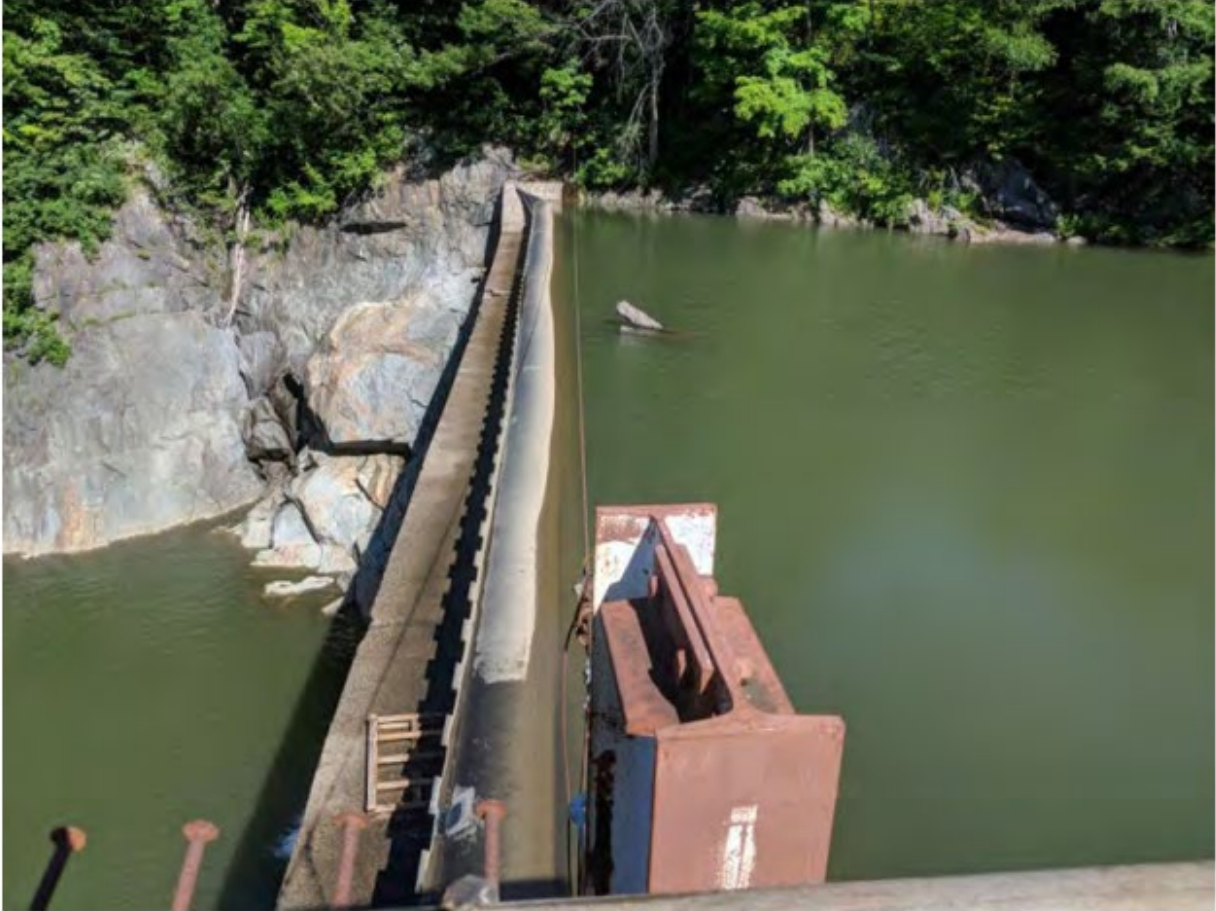
Figure 3. – Photograph of Bolton Falls Dam Spillway from top of left abutment.
