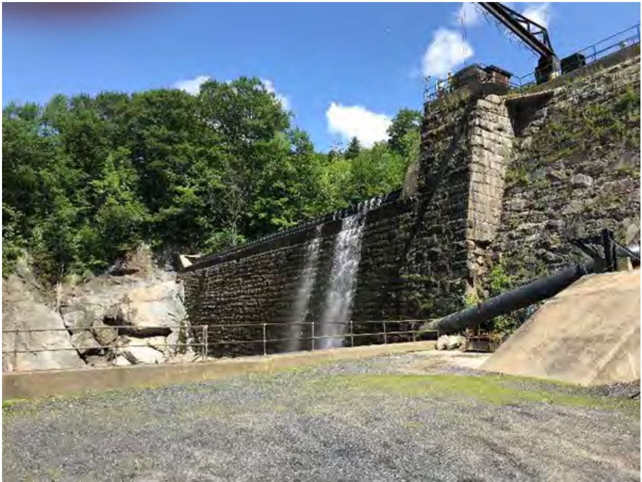
FIGURE A-1: PROJECT DAM AND BYPASS PIPE
