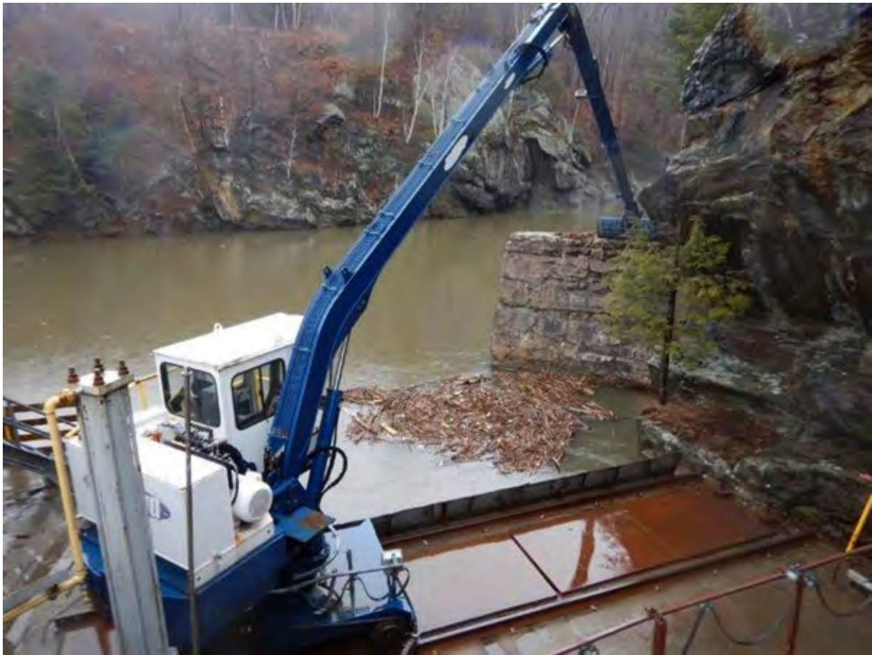
FIGURE A-3: POWERHOUSE INTAKE STRUCTURE AND TRASH RAKE
