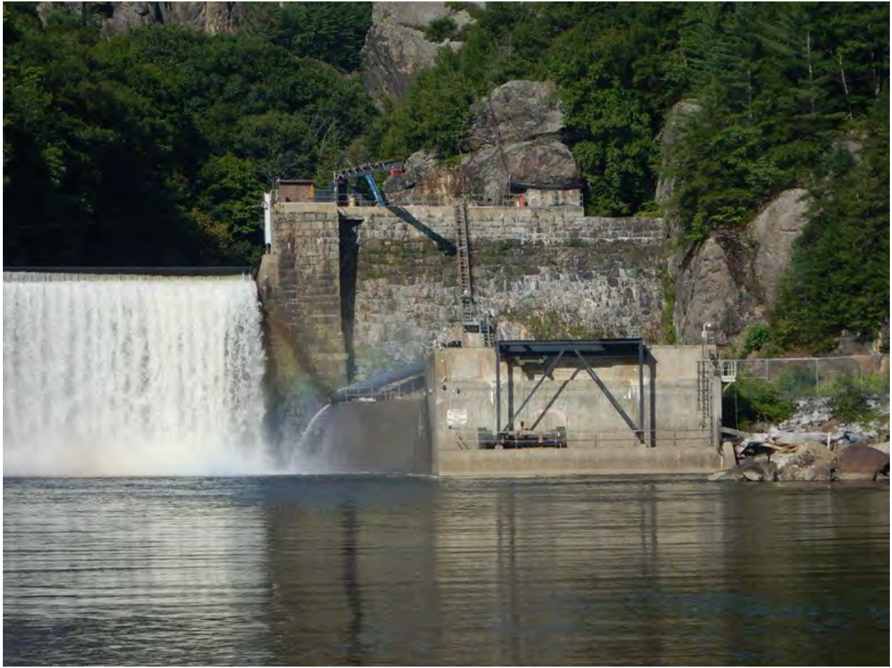
FIGURE A-2: PROJECT POWERHOUSE AND TAILRACE
