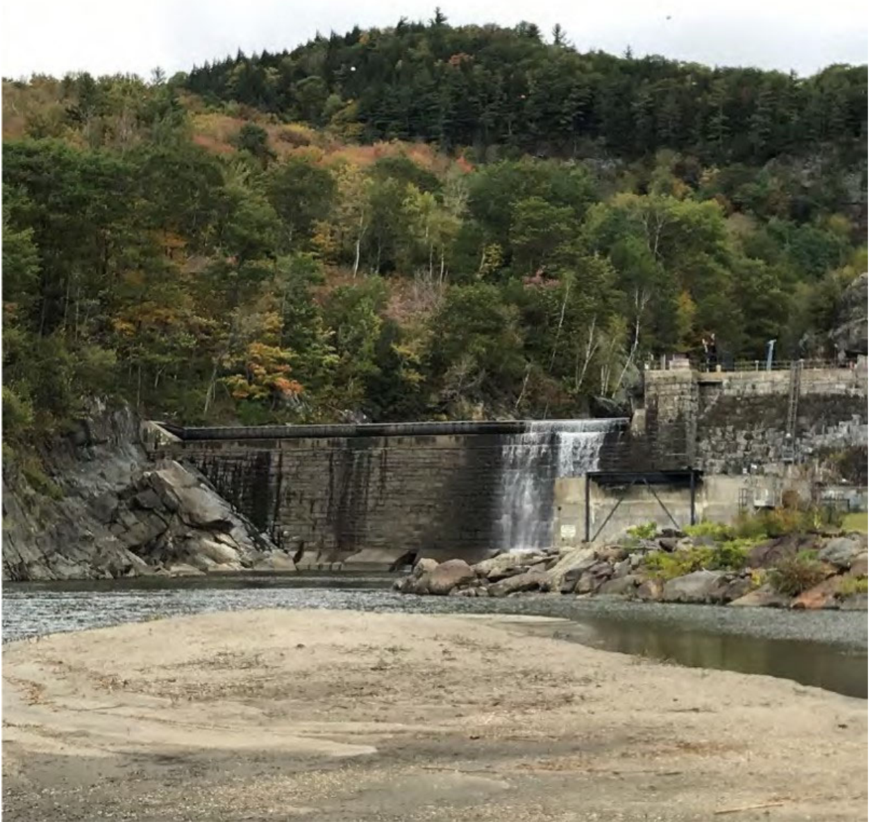
Photo E-2. View of the Bolton Falls Dam with a Spill Flow of 15 cfs. Source: license application.
