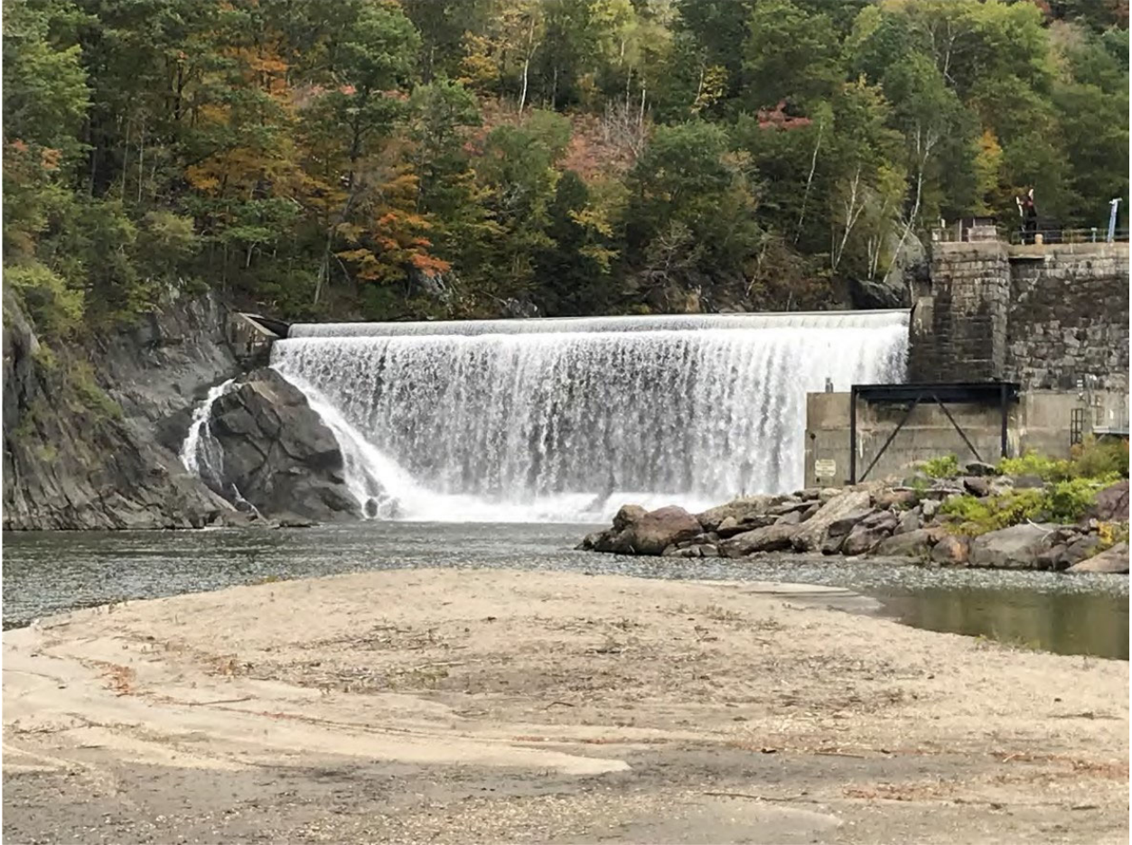
Photo E-5. View of the Bolton Falls Dam with a Spill Flow of 150 cfs. Source: license application.
