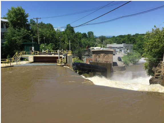
Figure 5 – Plant 9 Intake, Penstocks and Powerhouse
