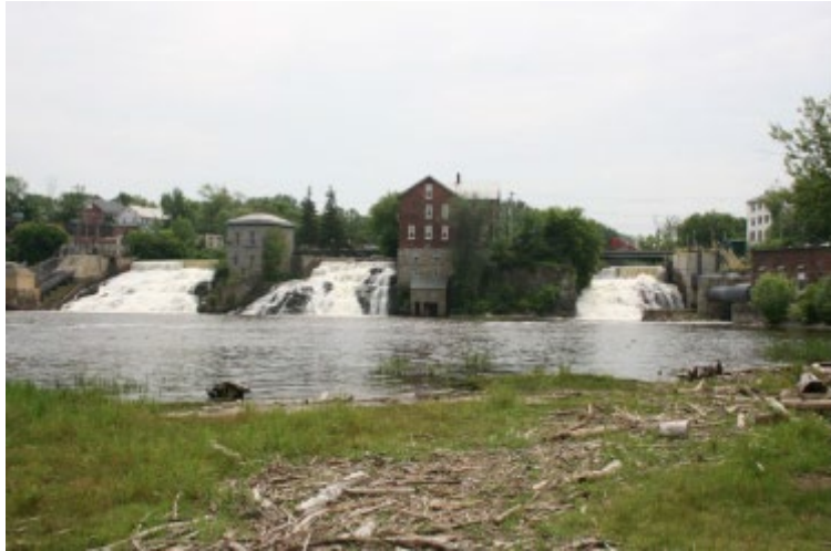
Figure 6 - Project Works (facing upstream)
