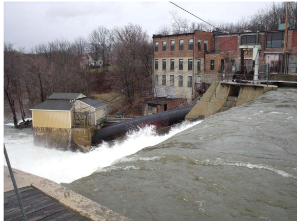
Figure 4 – Plant 9B Intake, Penstocks and Powerhouse
