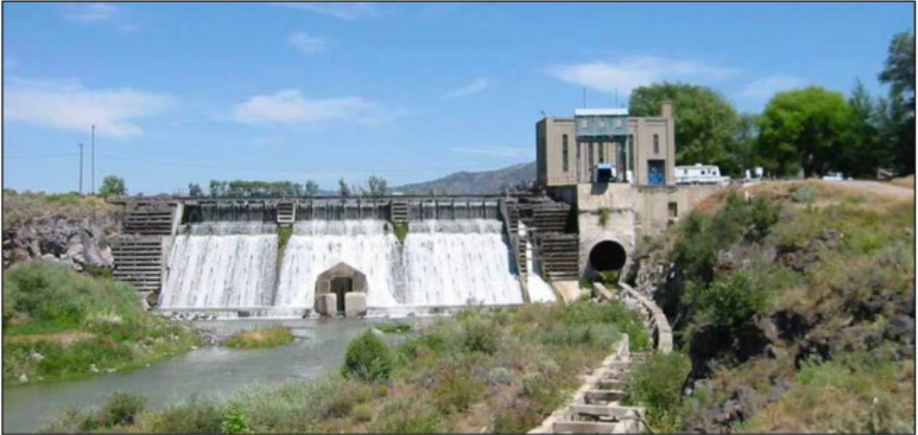
Figure 7. The Grace Dam of the Bear River Hydroelectric Project
