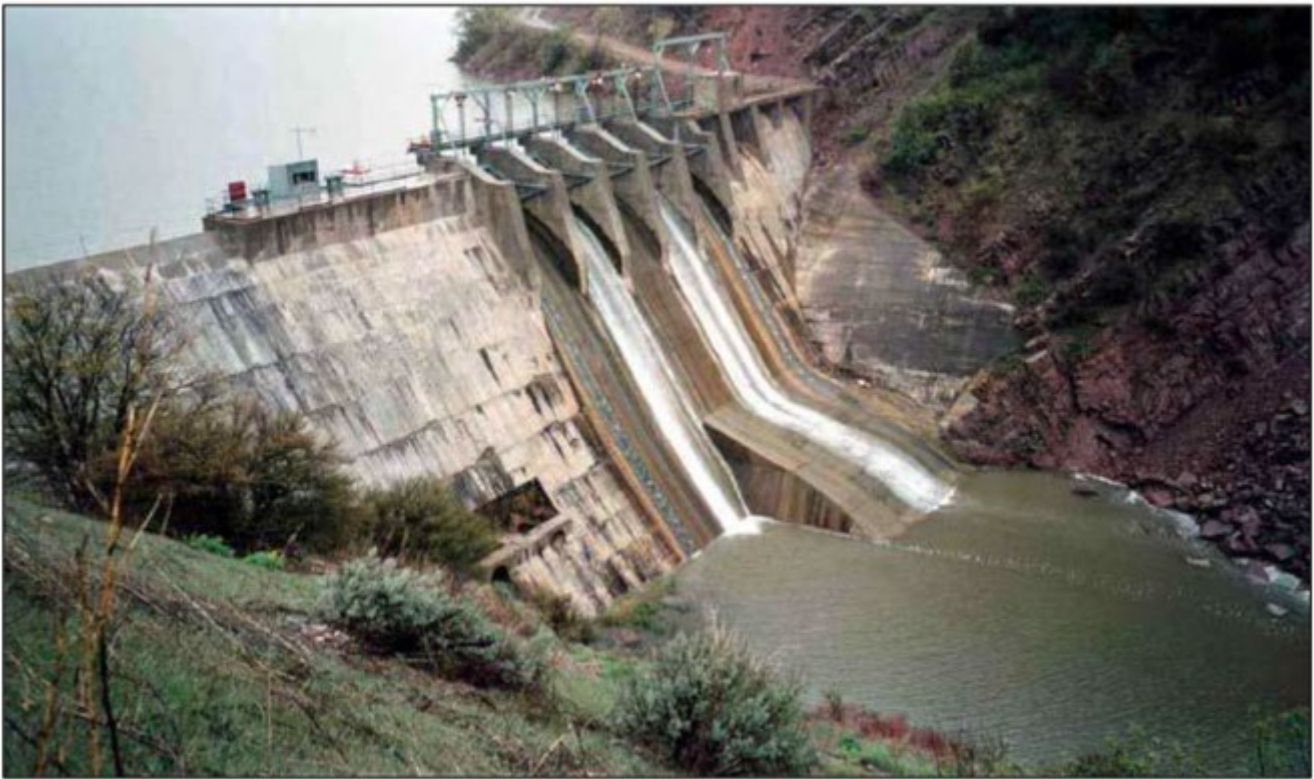
Figure 9. The Oneida Reservoir, Dam, and Spillway
