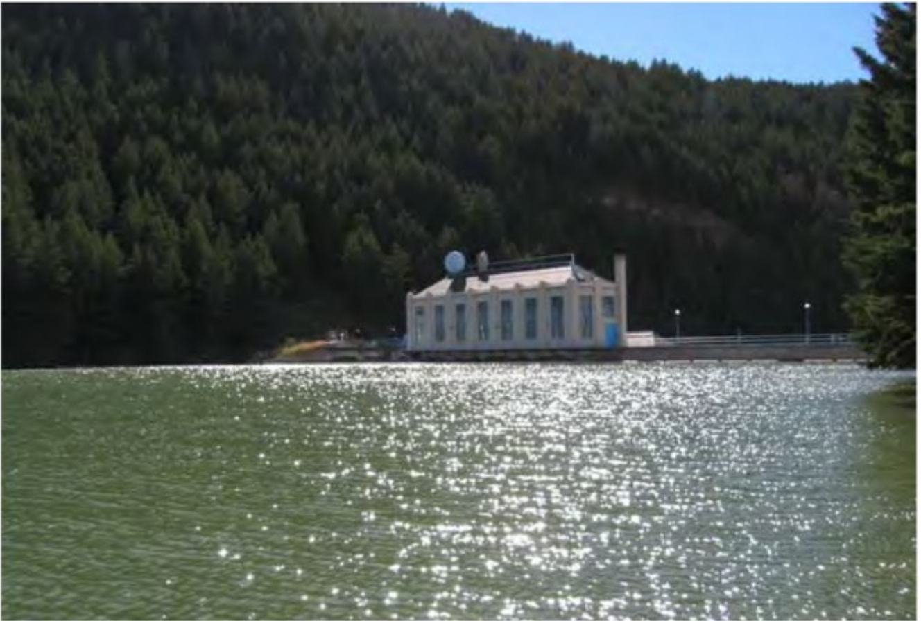
Figure 5. Soda Powerhouse and Alexander Reservoir
