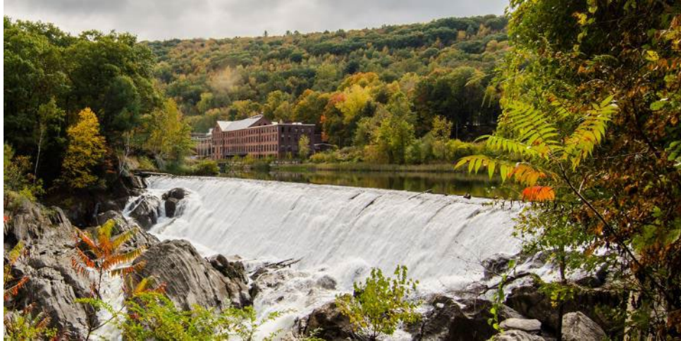
Figure 4 – North Dam Looking West
