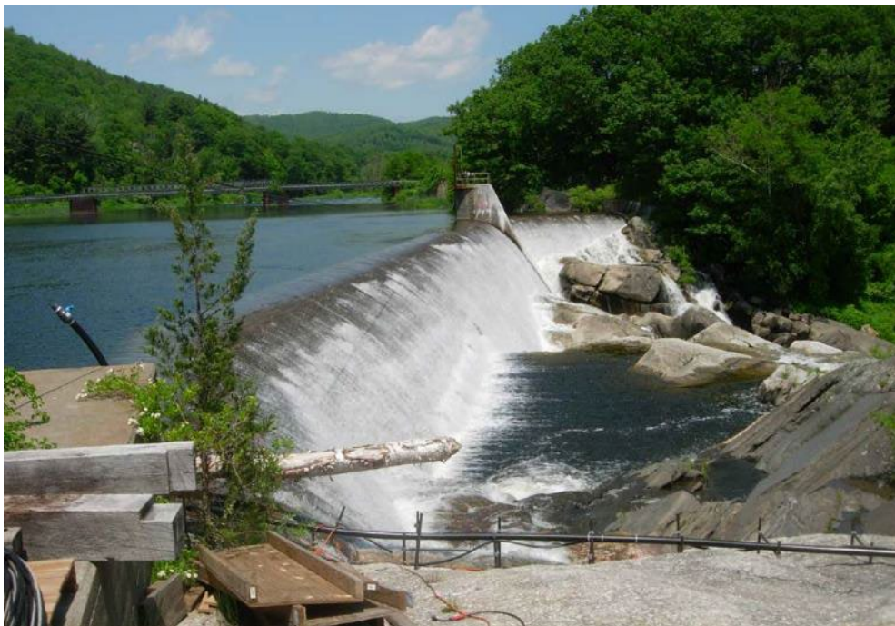
Figure 5 – South Dam Looking East and Upstream
