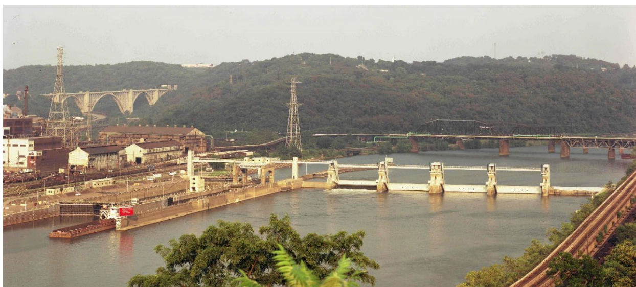
Figure 2 – ACOE Braddock Lock and Dam
