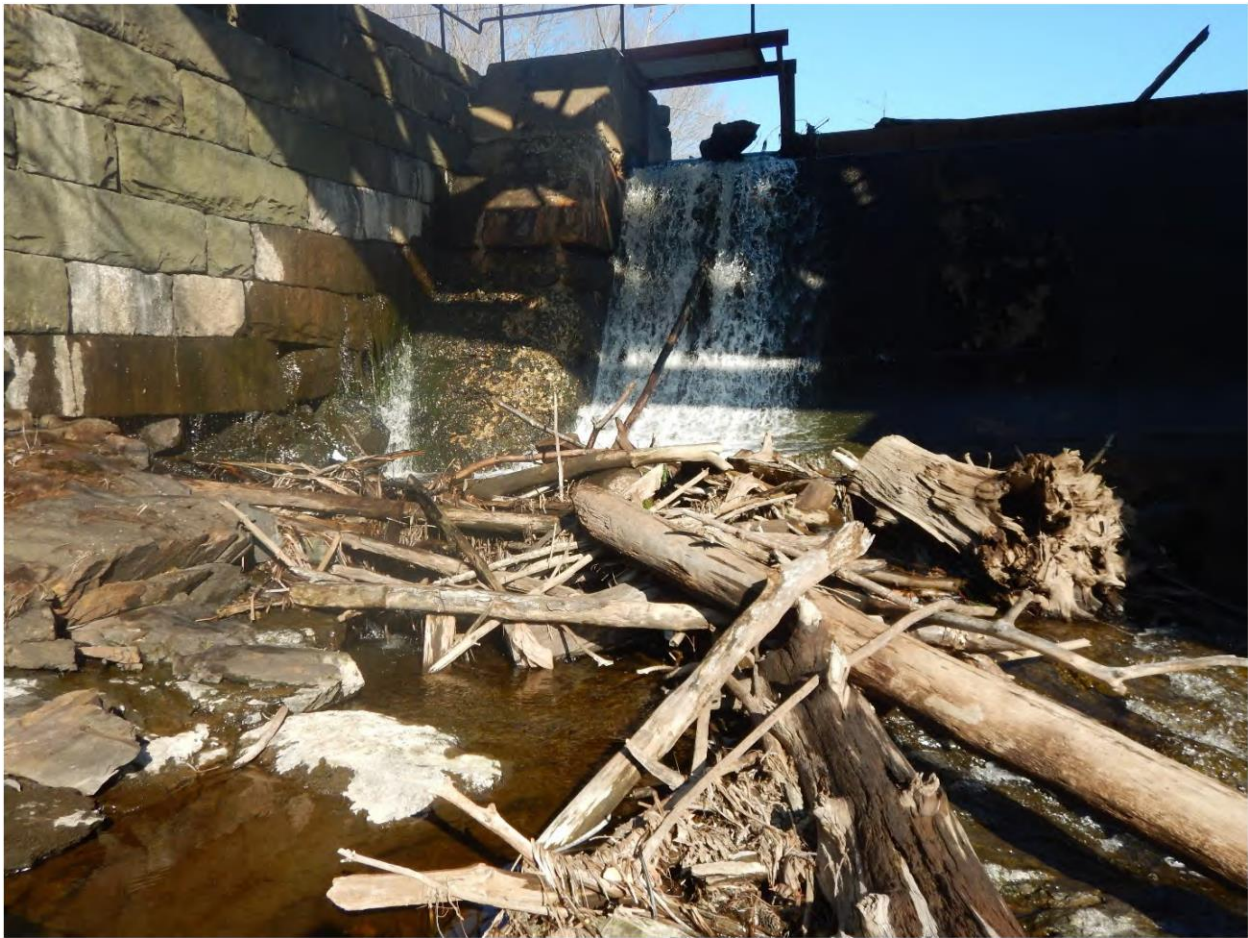
Figure 10. Debris piled immediately downstream of the dam on the river right (Source: The Town, 2019).
