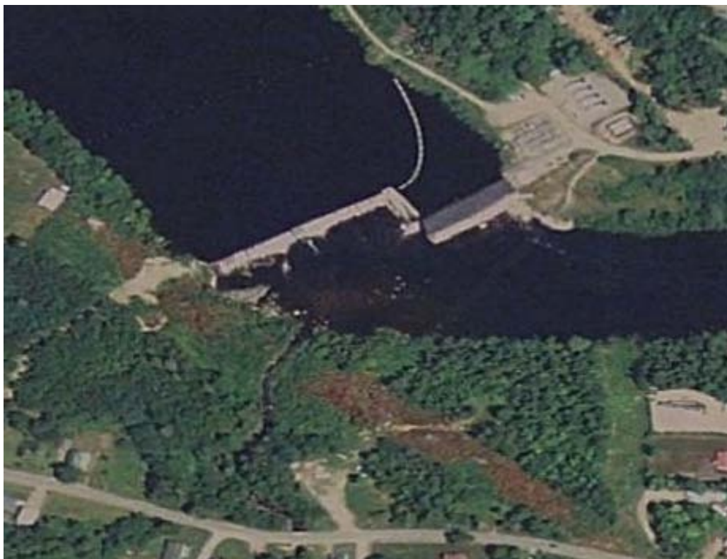
Figure 4-28. Aerial view of the Medway Hydroelectric Project.
