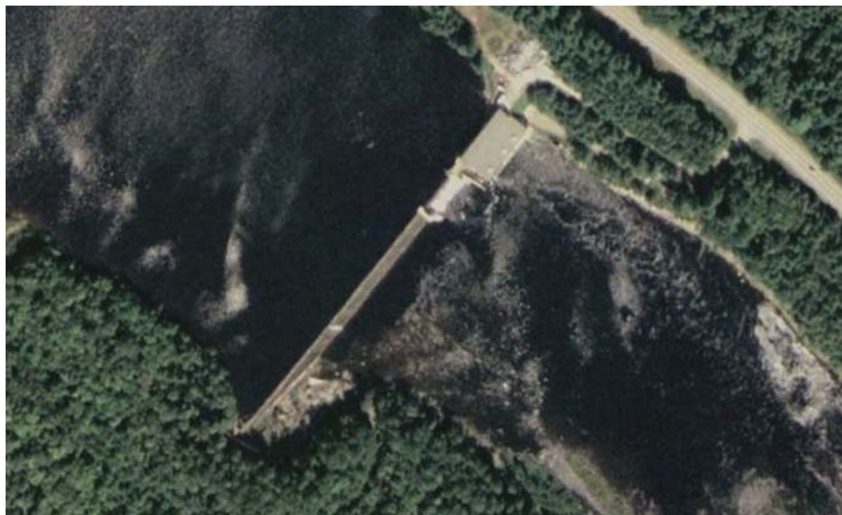
Figure 4-15. Aerial view of the Mattaceunk Hydroelectric Project.
