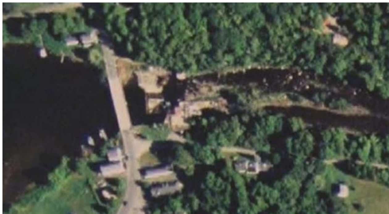
Figure 4-46. Aerial view of the Sebec Hydroelectric Project.
