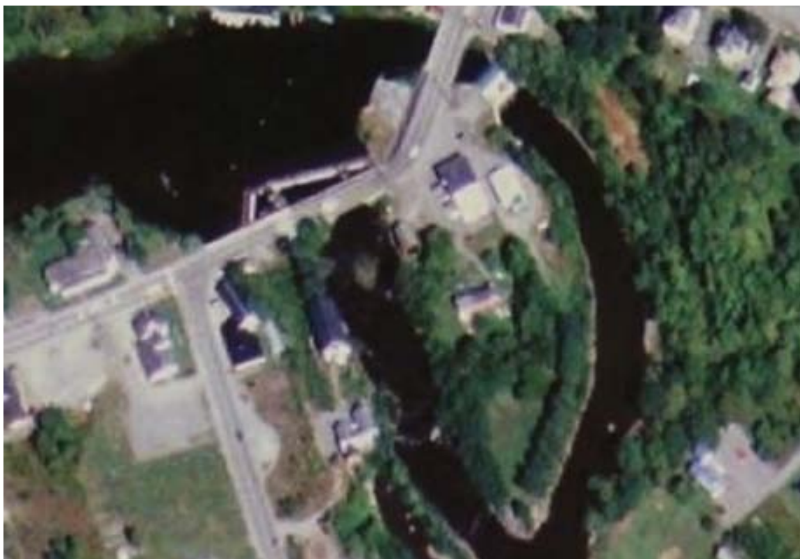
Figure 4-43. Aerial view of the Milo Hydroelectric Project.
