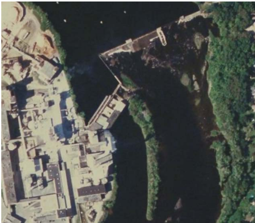
Figure 4-4. Aerial view of the Great Works Hydroelectric Project.
