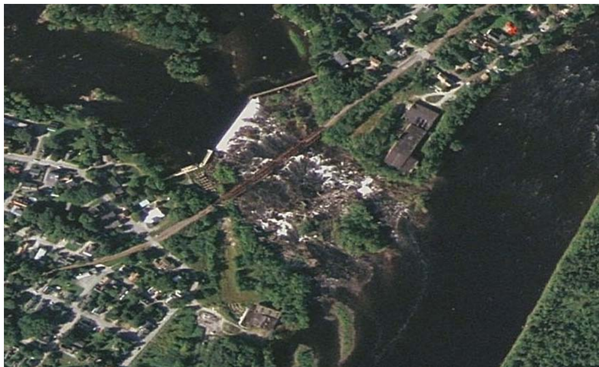
Figure 4-18. Aerial view of the Orono Hydroelectric Project.
