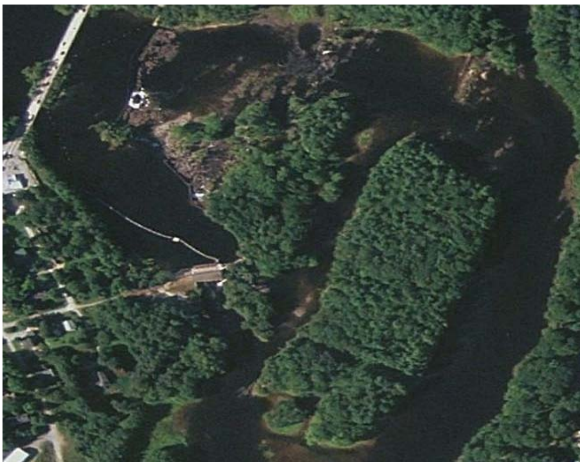
Figure 4-23. Aerial view of the Stillwater Hydroelectric Project.
