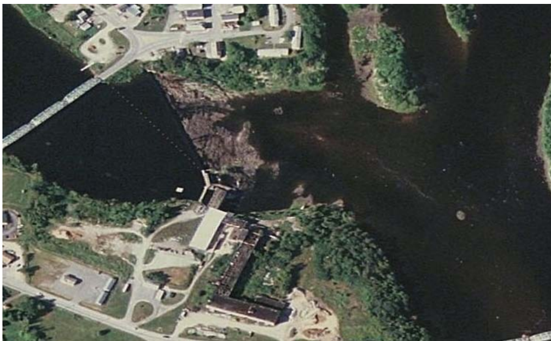
Figure 4-31. Aerial view of the Howland Hydroelectric Project.
