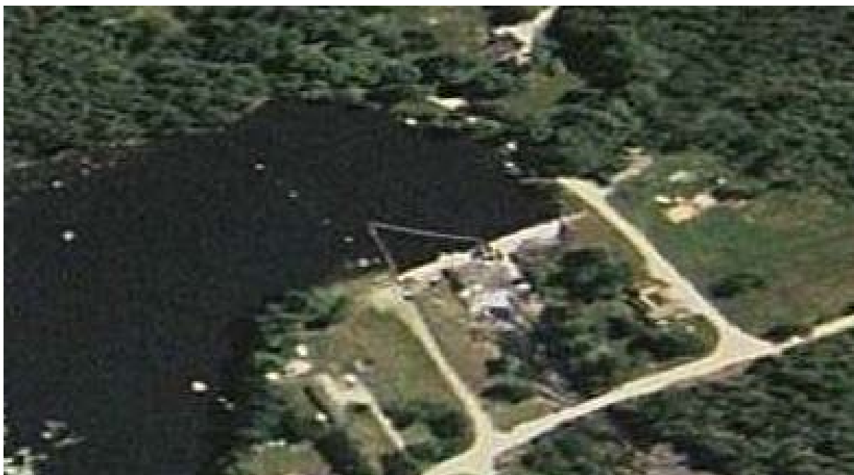
Figure 4-37. Aerial view of the Lowell Tannery Hydroelectric Project.
