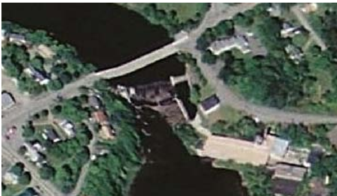
Figure 4-34. Aerial view of the Brown's Mill Hydroelectric Project.
