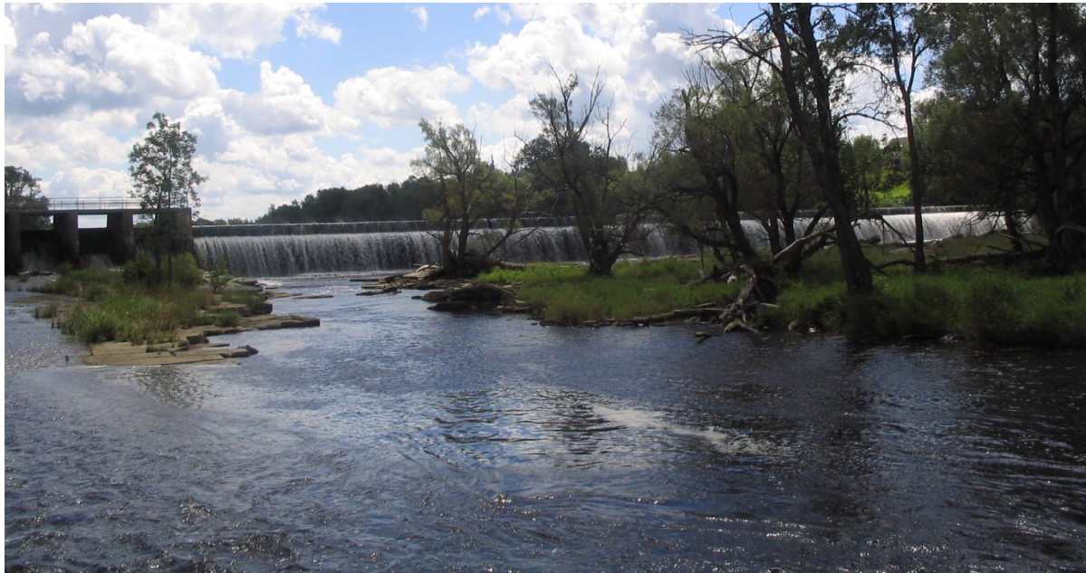
Figure 2. The Deferiet dam, with 3-foot pneumatic flashboards
