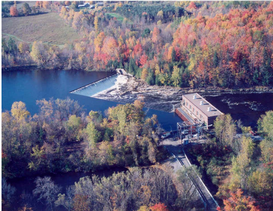
Figure 1. Powerhouse and L-shaped dam at the Herrings Development.
