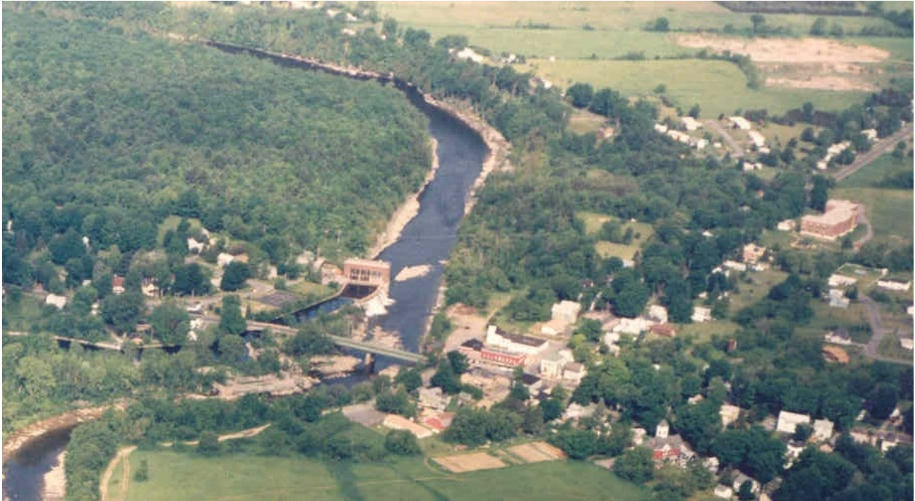
Figure 3. Downstream view of power canal and bypassed reach at the Kamargo Development.
