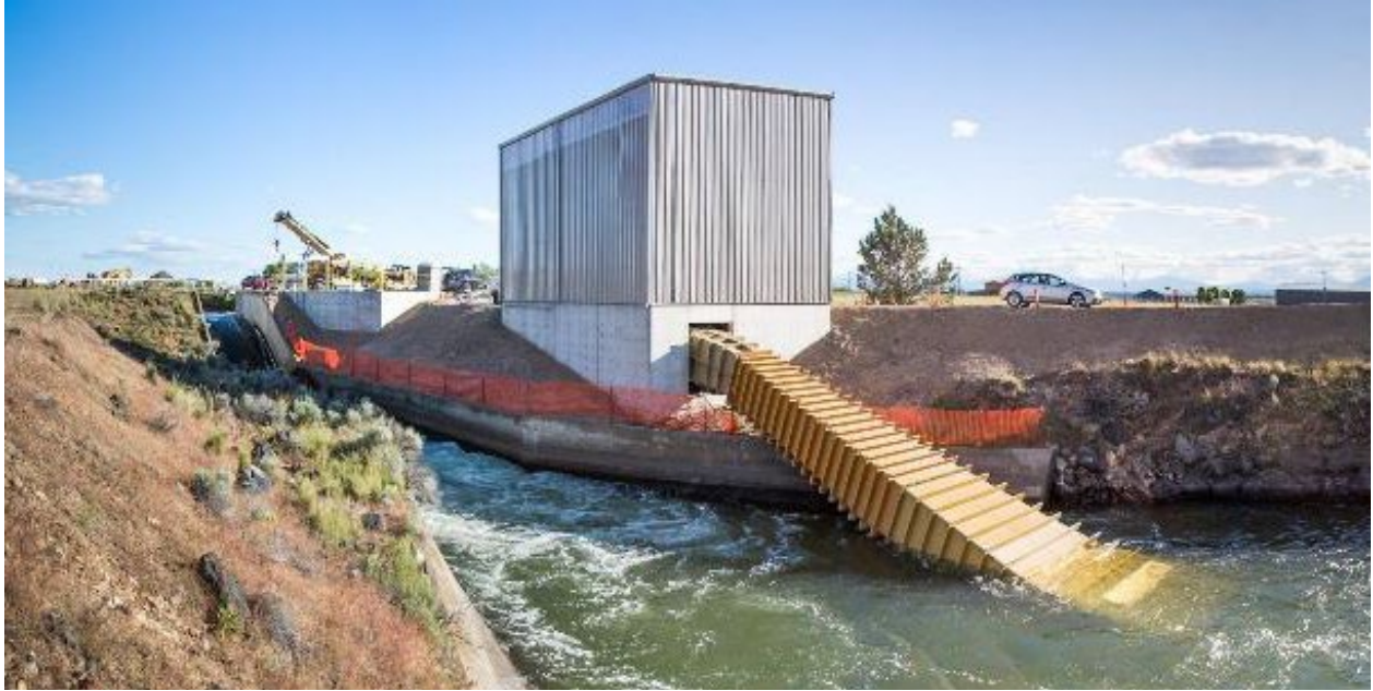
Figure 4. Powerhouse, tailrace, and draft tube
