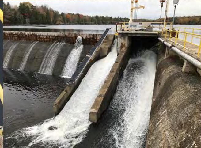
M3: DS Bypass Sluice
