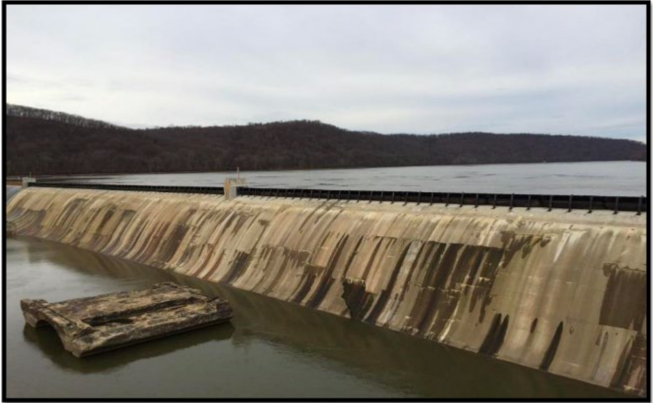
Figure 4. Holtwood Dam and Obermeyer Gates
