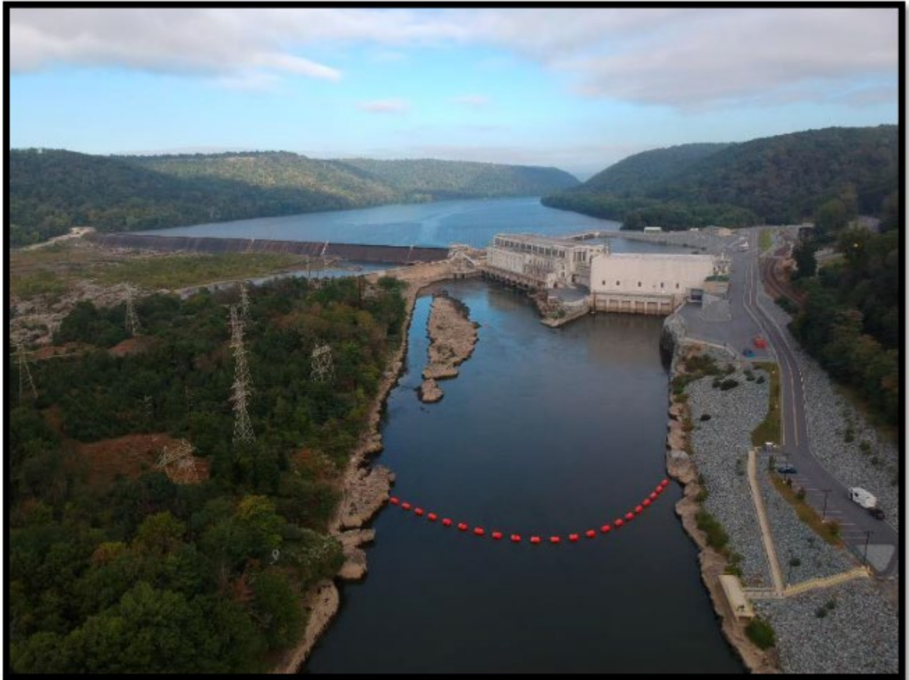
Figure 6. Holtwood Project Features with Powerhouses and Tailrace on right
