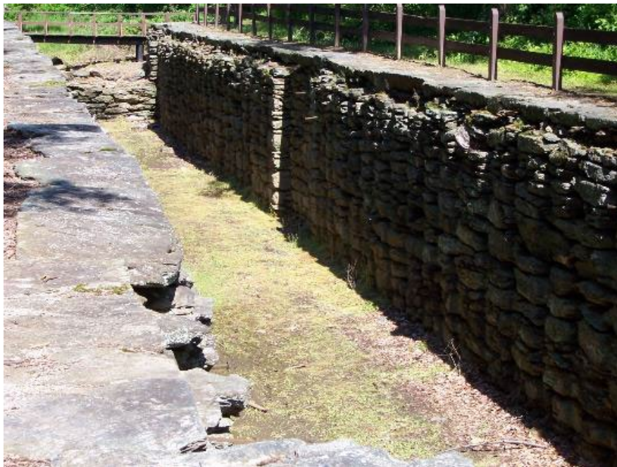
Figure 13. Preserved walls of Lock No. 12 of the Susquehanna and Tidewater Canal system
