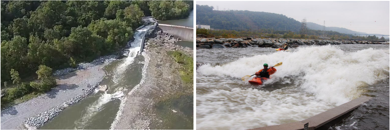
Figure 16. Whitewater facility on west shore of dam and whitewater boater (Sources: https://vimeo.com/111790402 and https://www.americanwhitewater.org/content/Project/view/id/5/ )
