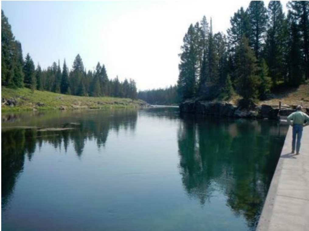
Figure 7 – Impoundment of the Buffalo River
