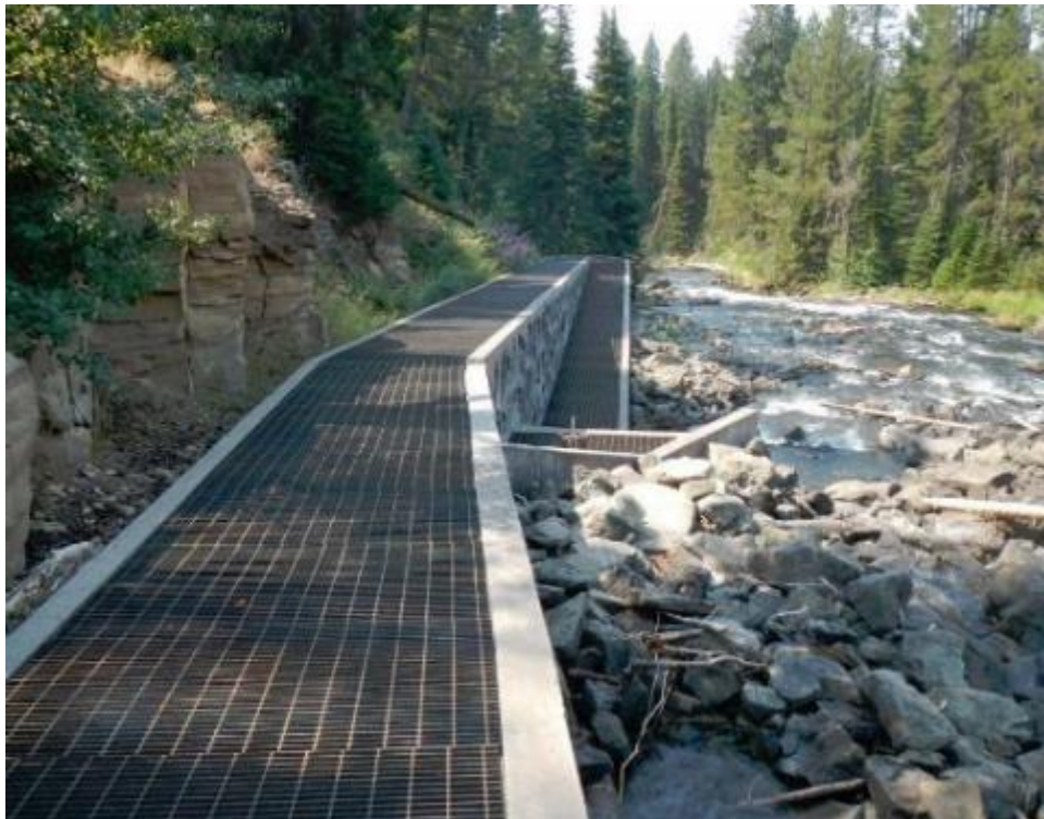
Figure 6 – Looking downstream from spillway at bypass and fishway
