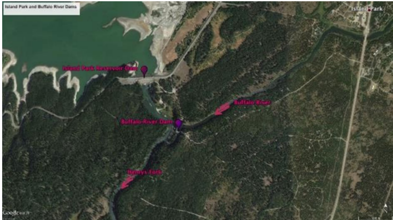
Figure 2 – Aerial Showing the Buffalo River and Island Park Dams
