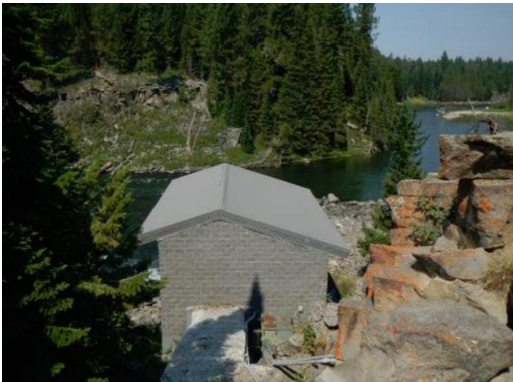
Figure 8 – Powerhouse and Henry's Fork looking upstream
