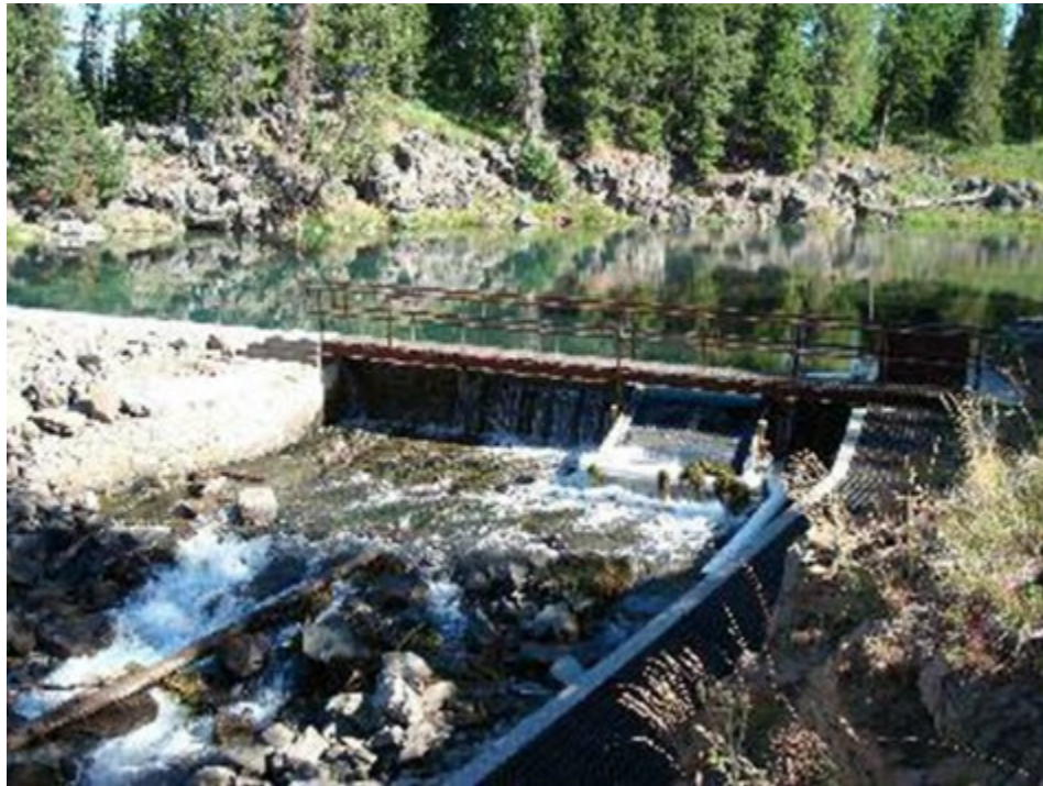
Figure 5 – Looking upstream at spillway with showing bypass and fishway along east (left) bank of river
