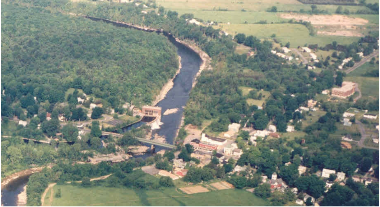
Figure 3. Downstream view of power canal and bypassed reach at the Kamargo Development.
