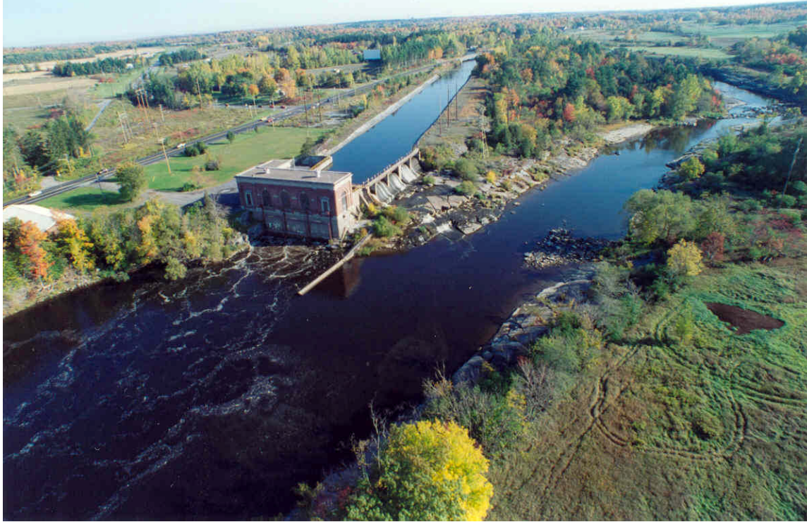
Figure 4. Upstream view of tailrace, powerhouse, canal, and bypassed reach at the Black River Development.
