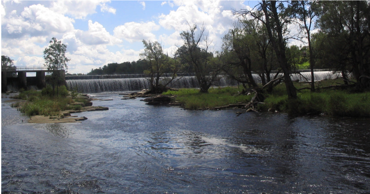
Figure 2. The Deferiet dam, with 3-foot pneumatic flashboards
