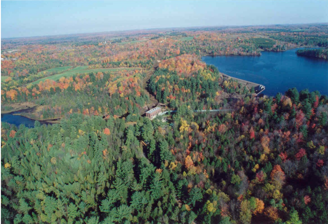
Photo 10. Powerhouse and dam at High Falls Development.
