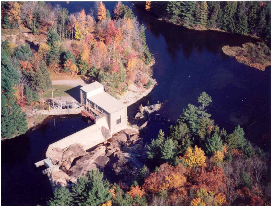
Photo 6. Powerhouse and dam at Elmer Development.
