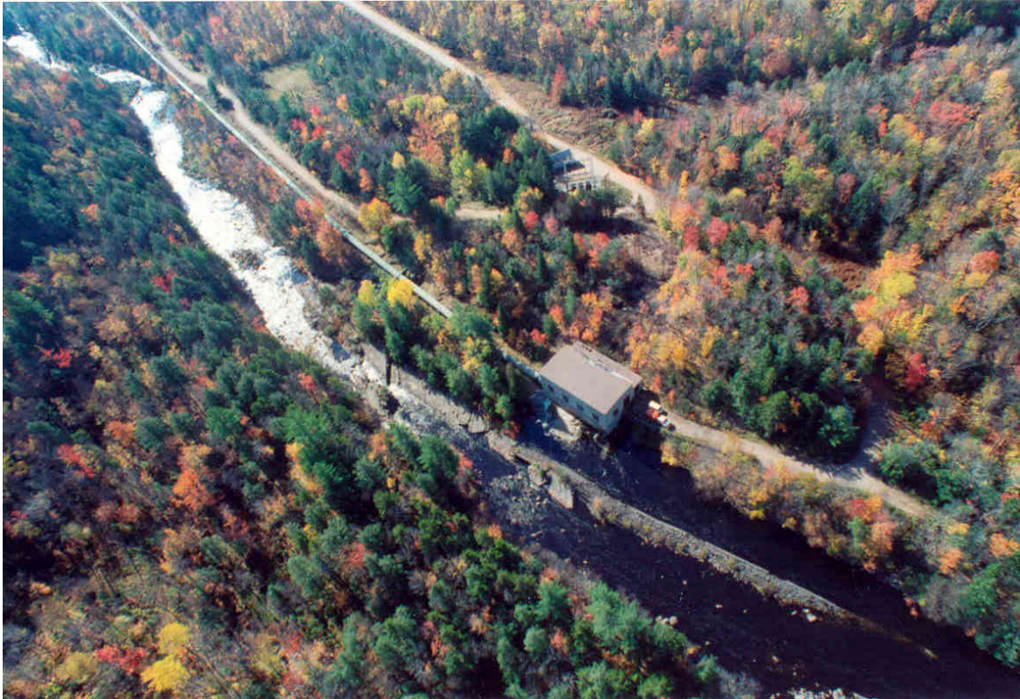
Photo 3. Powerhouse at Eagle Development.
