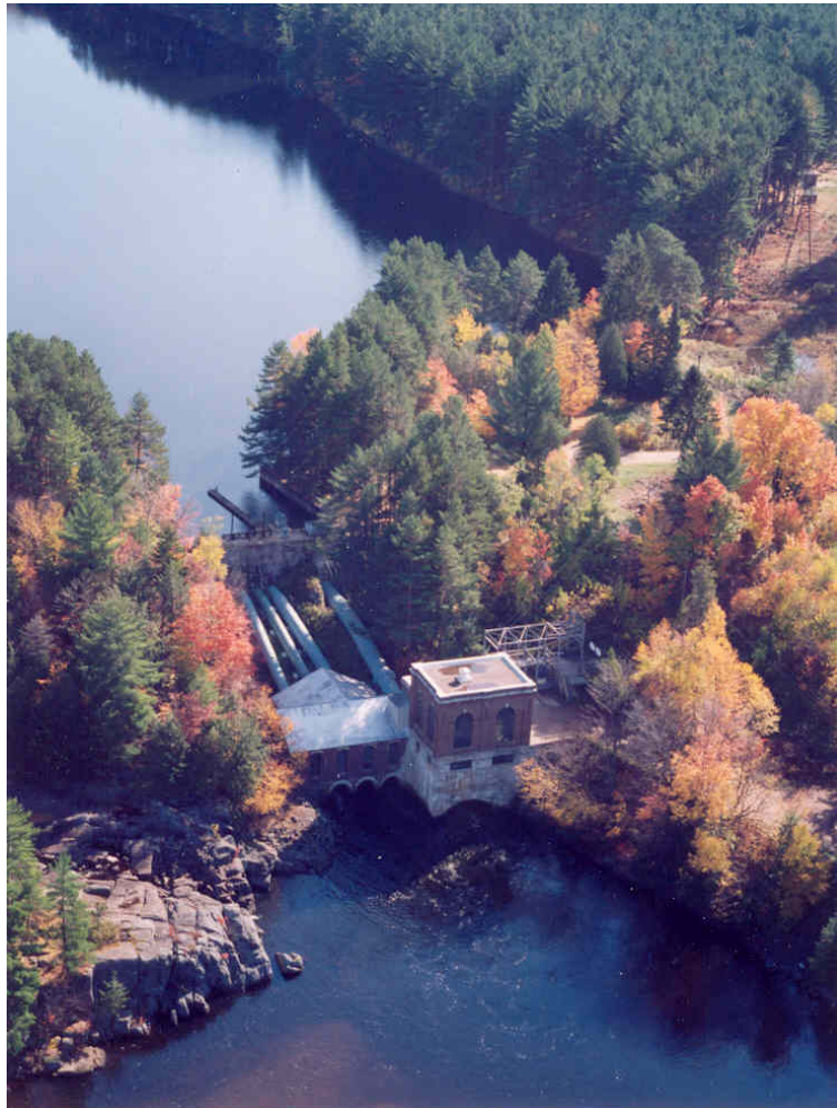
Photo 5. Powerhouse at Effley Development.
