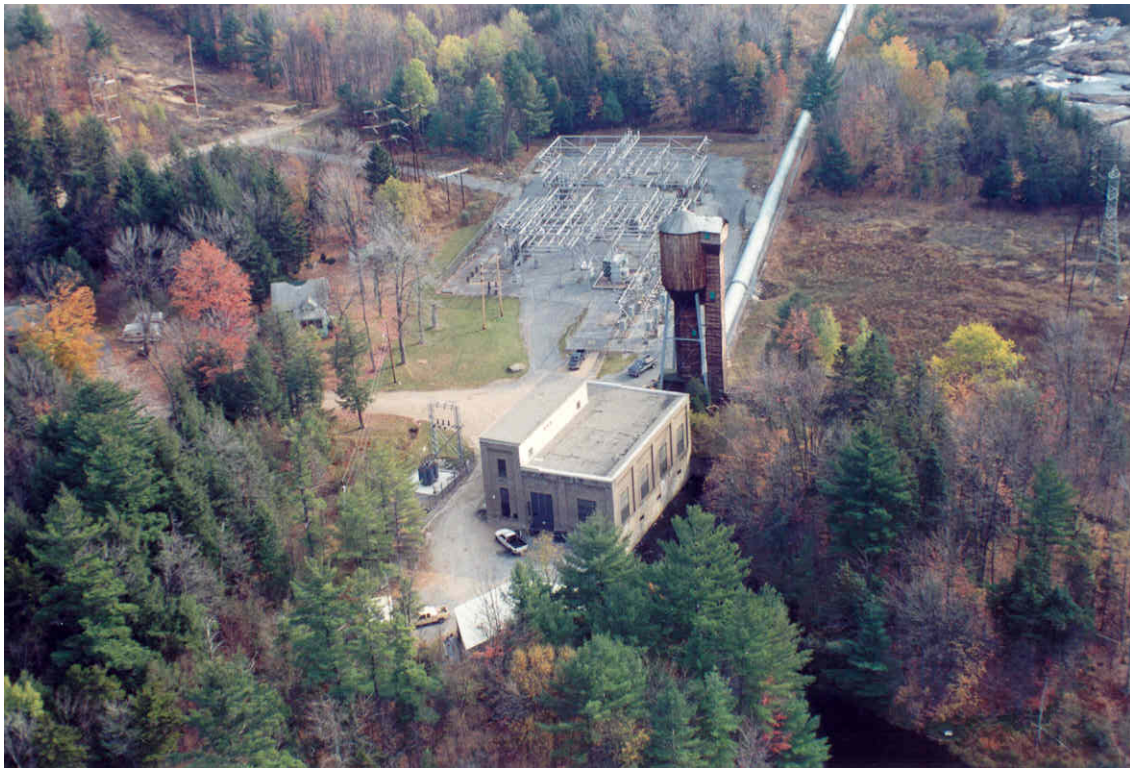
Photo 7. Powerhouse and surge tank at Taylorville Development.
