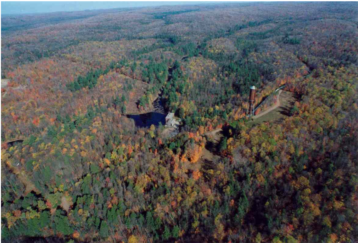
Photo 1. Powerhouse and surge tank at Moshier Development.
