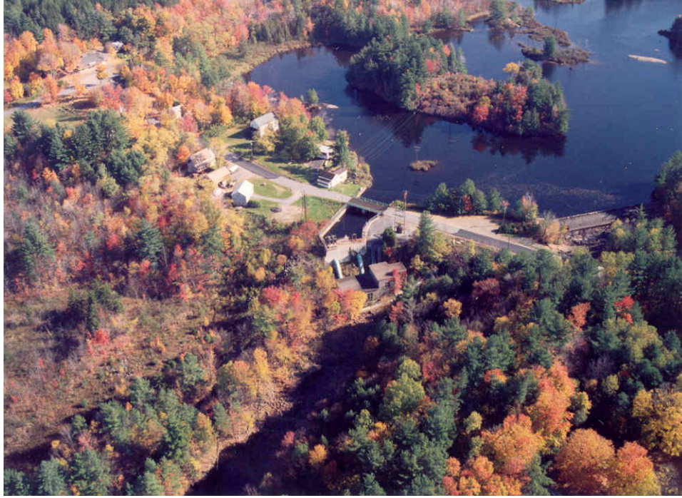
Photo 9. Powerhouse and dam at Belfort Development.
