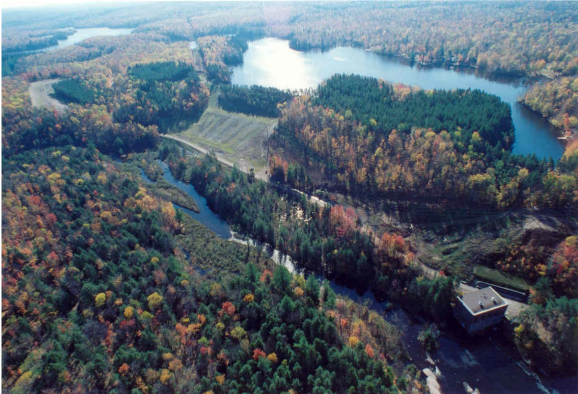
Photo 4. Powerhouse at Soft Maple Development.
