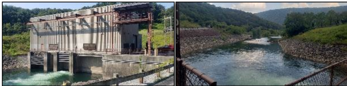
Figure 3-Powerhouse (left) and Tailrace (right)
