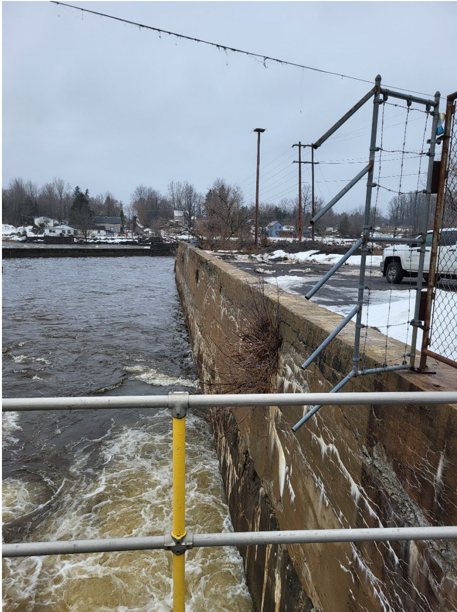
Photo 9 Shoreline Access at Dam 18 (Beanery)
