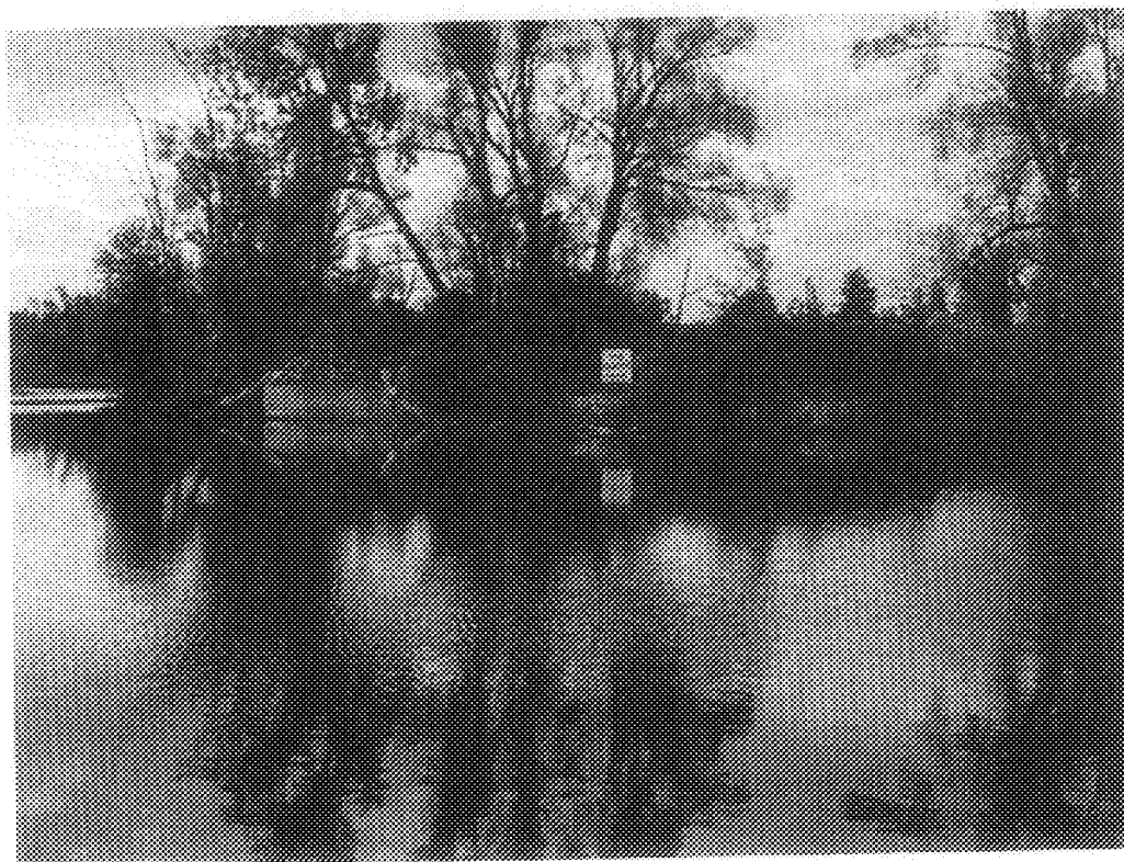
Photo No. 9 - View of upstream warning sign on Papermill Island upstream of Dam No. 17.
