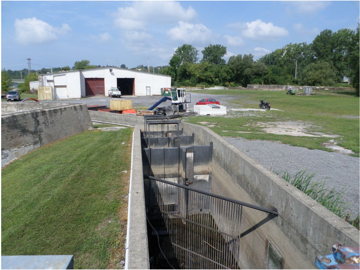
Photo 6 Fish Ladder at Dam 18
