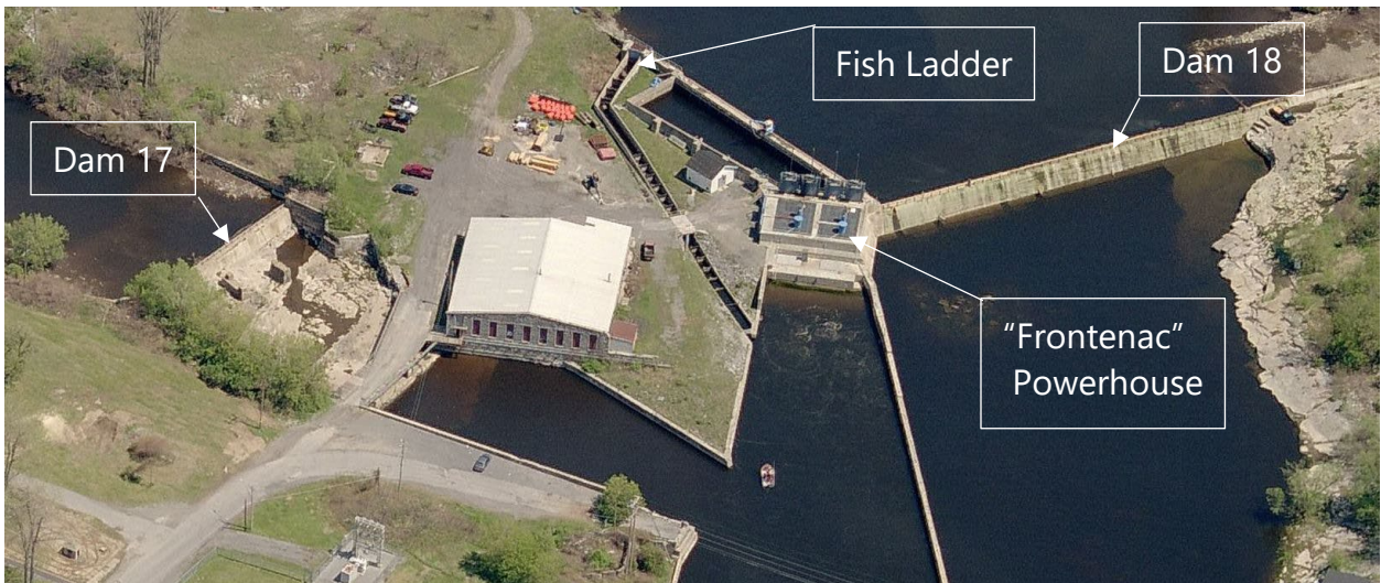
Photo 5 Aerial View of the Dexter Project's "Frontenac" powerhouse (river right of Dam 18) and Appurtenant Facilities
