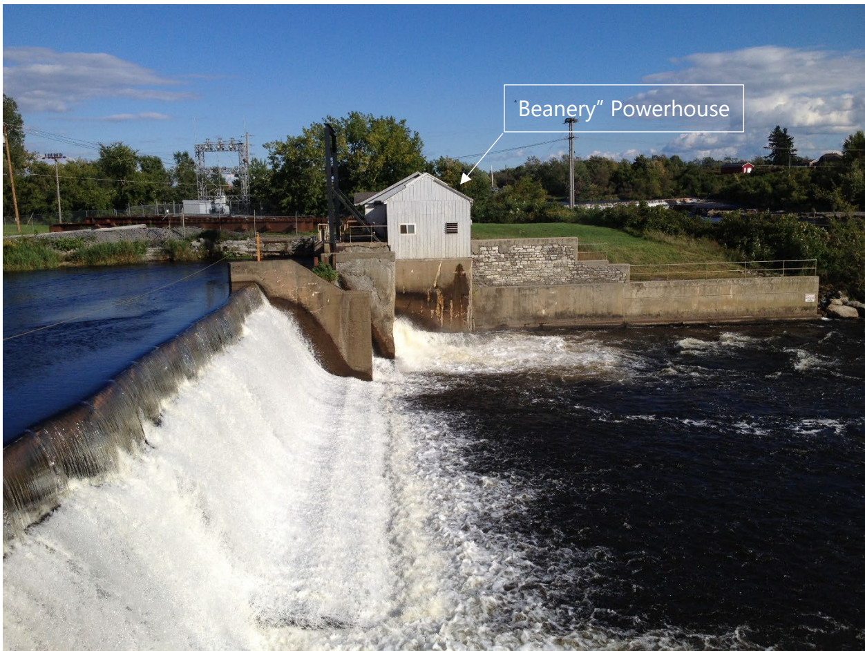
Photo 3 Dexter Project's "Beanery" Dam 16, spillway looking from "Main" powerhouse
