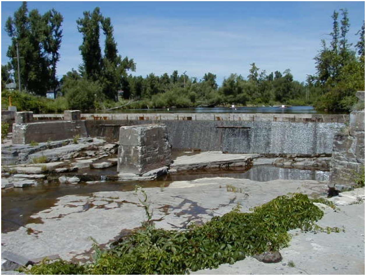
Photo 4 Dexter Project's Dam 17
