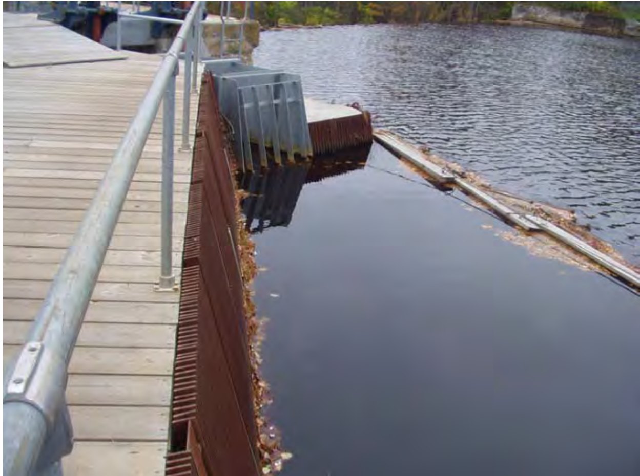
FIGURE A-6: DENIL FISH LADDER EXIT/ENTRANCE TO DOWNSTREAM FISH PASSAGE FACILITY
