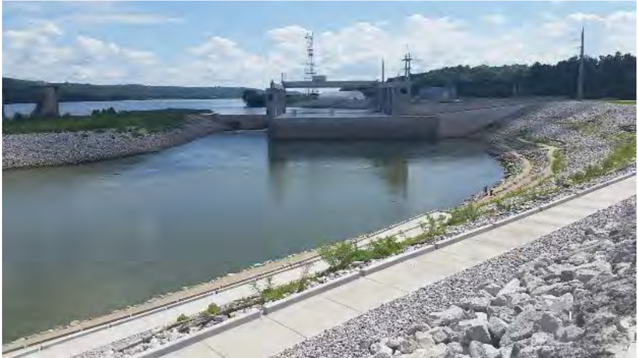
Photo 6 – View of Project Tailrace Channel
