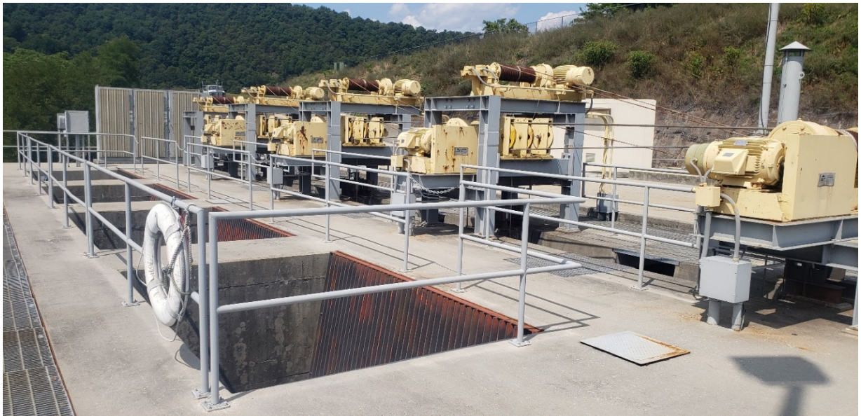
Figure 6. Intake trash racks and temperature control equipment
