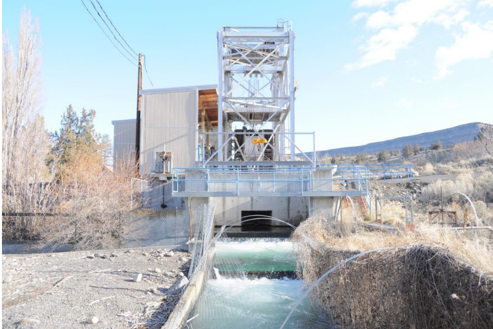
Figure 7. Pelton adult fish trap with view of jump pool.
