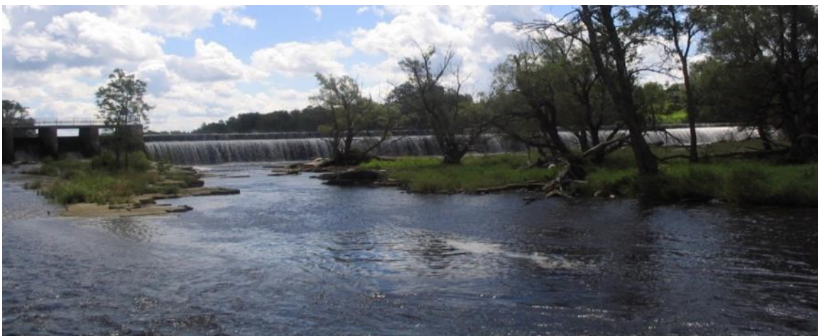
Figure 2 - The Deferiet dam, with 3-foot pneumatic flashboards
