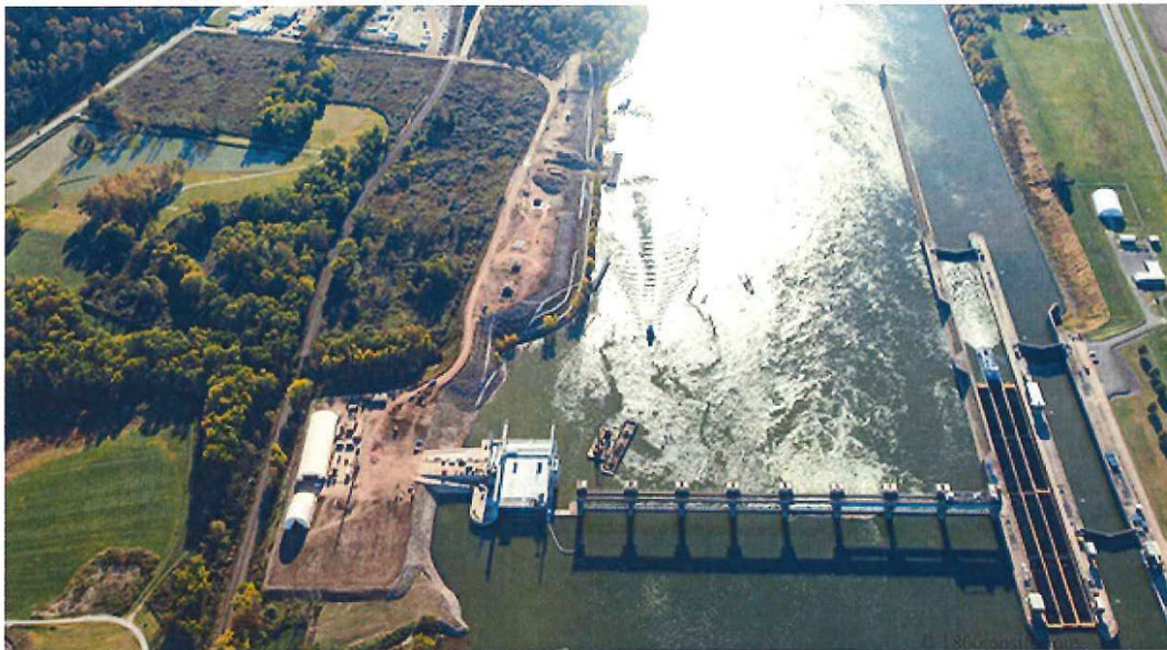
Figure 3. View of Project looking downstream.
